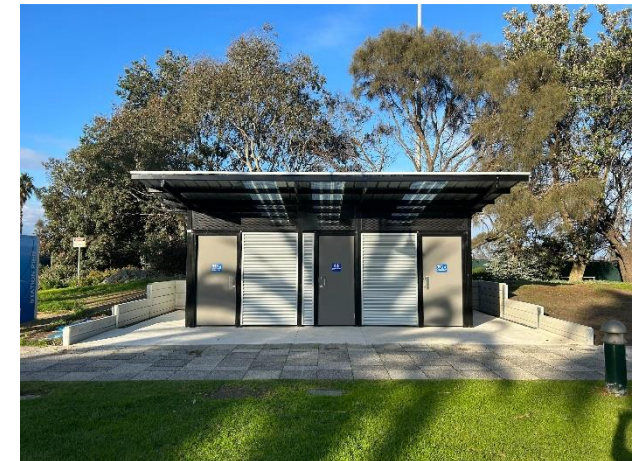
New public toilets at Waterfront Place
