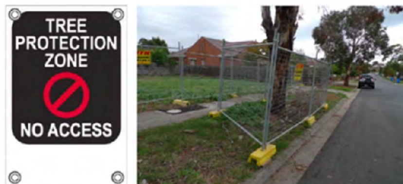
Figure 7: Example of signage for TPZ and of appropriate TPZ fencing for a street tree that can be utilised for all retained trees.
