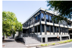
Late 20 century office building
