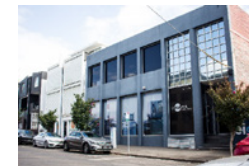
Mixed use SOHO building
