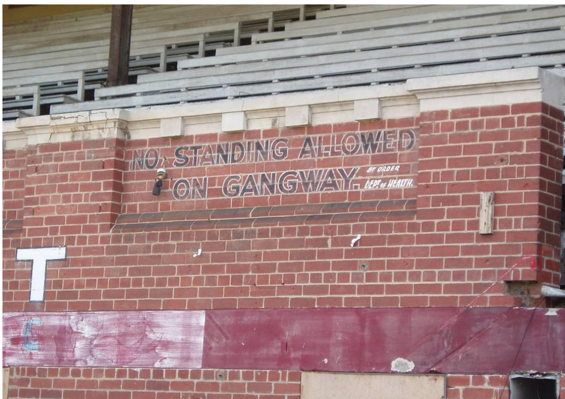
Figure 9 South Melbourne Grandstand, showing early painted signage and original timber seating.
