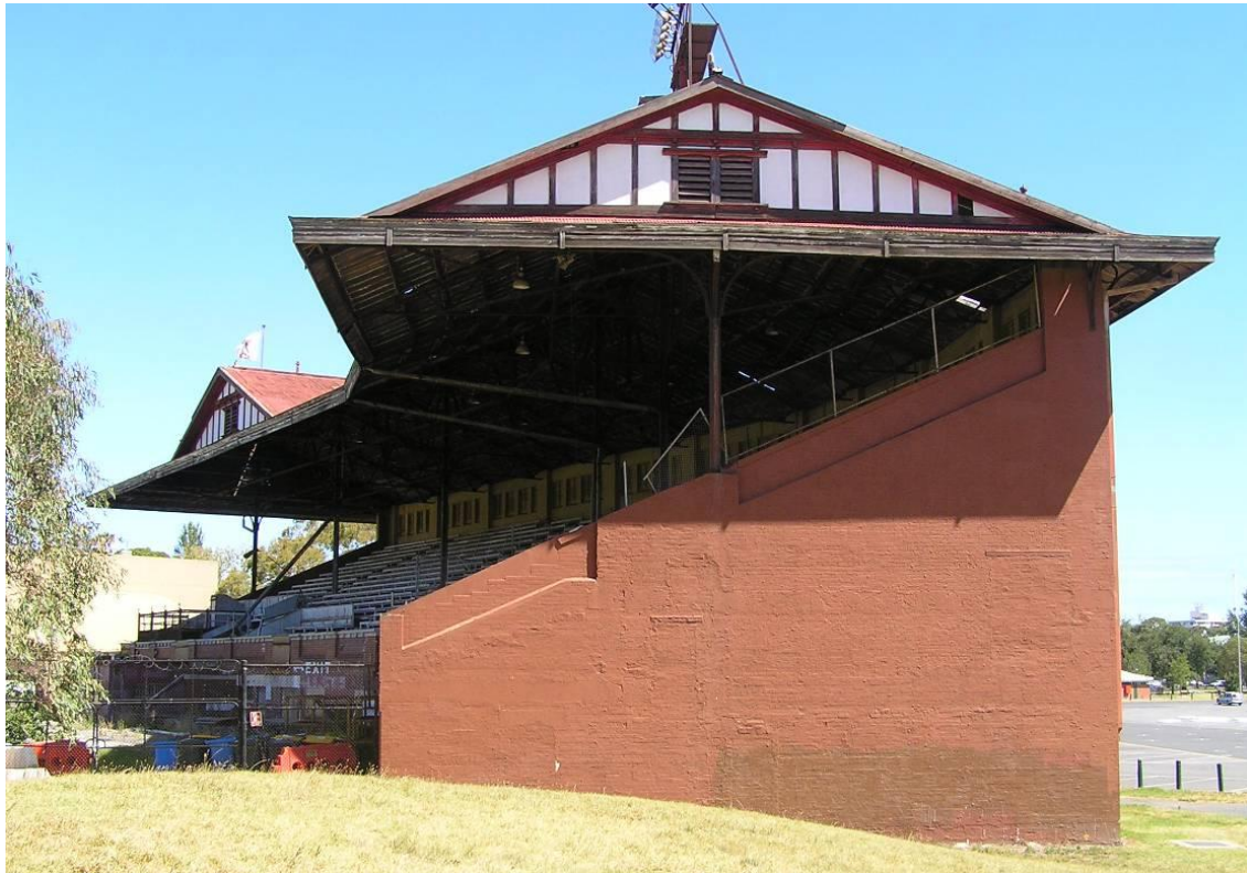
Figure 8 The South Melbourne Cricket and Football Club Grandstand, (1926-28) showing distinctive cranked form and open roof carried over trusses with gable ends.
