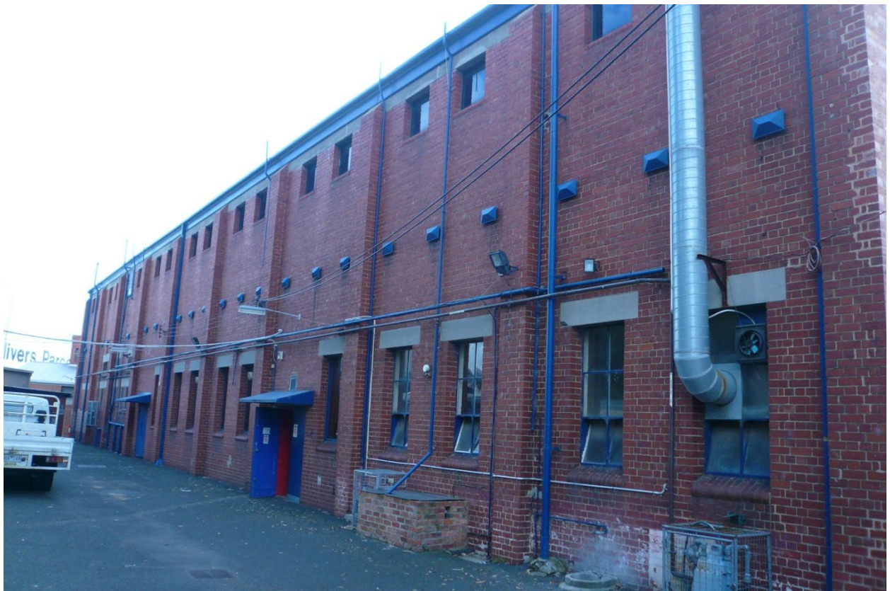
Figure 7 Rear elevation showing unpainted brick and render finishes.
