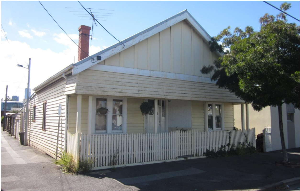
Figure 9 Atypical early 1920s timber bungalow at 234 Bridge Street.
