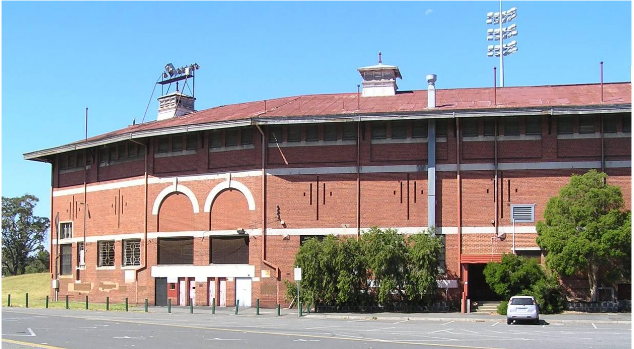
Figure 10 The west elevation of the South Melbourne Grandstand, showing row of highlight windows beneath the eaves.
