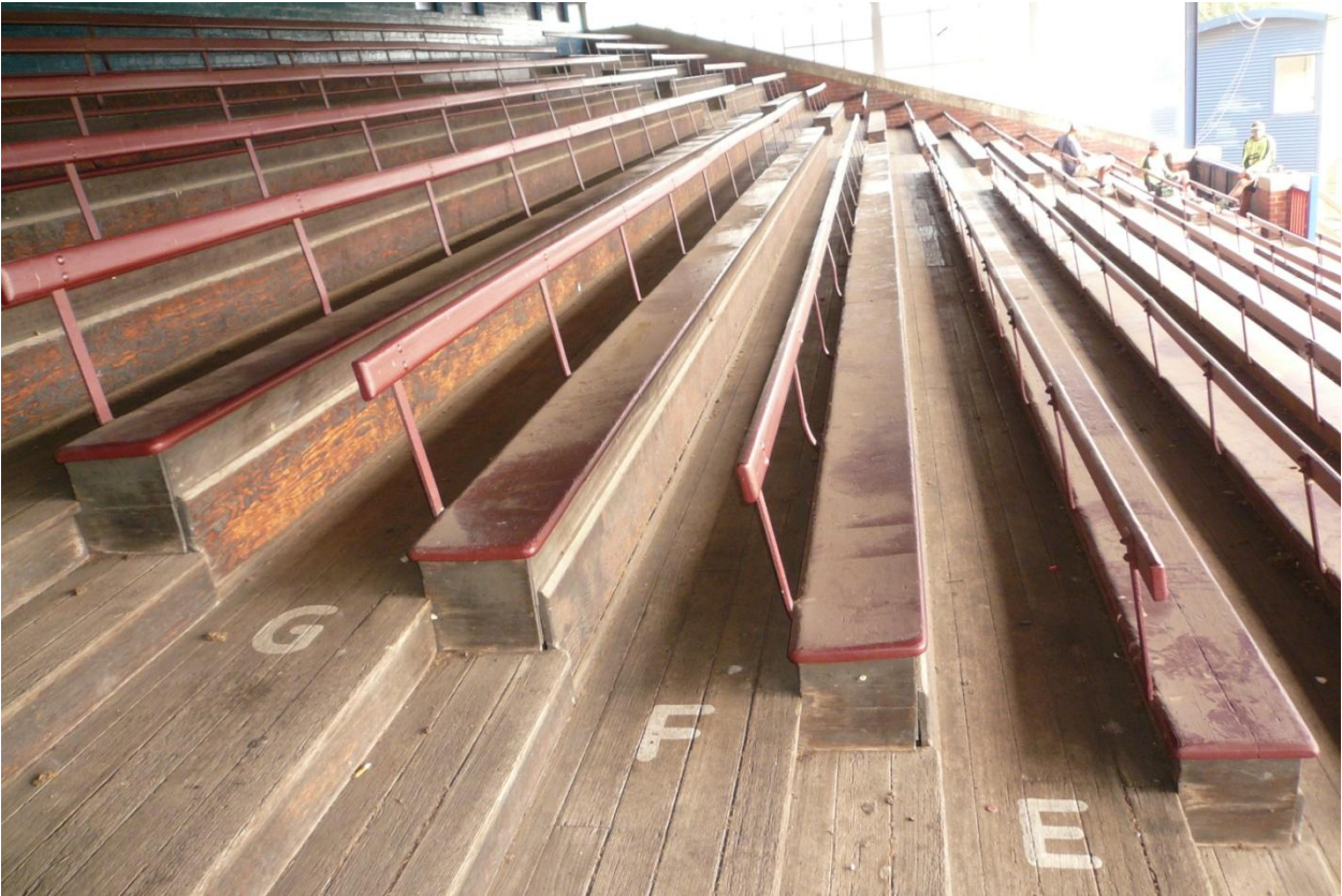
Figure 5 Timber seating plats and painted row identifiers.
