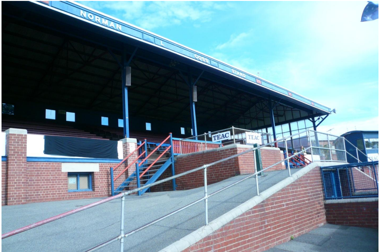
Figure 6 Entry ramp and access stairs, Norman L Goss Stand.
