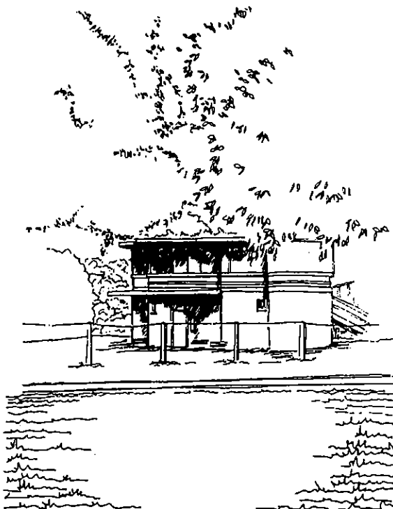
FIGURE 22.0 Harry Trott Pavilion Both the Harry Trott Pavilion and the Ross Gregory Pavilion are old concrete block houses with extensions added in a piece-meal fashion.
