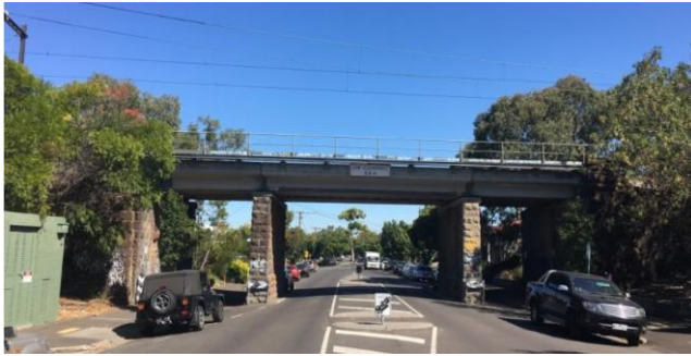
Grosvenor Street bridge
