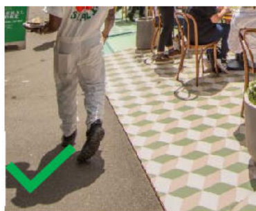
Figure x: A mat creates a flush transition from the platform to the footpath.
