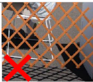
Figure x: Flimsy materials like lattice should not be used
