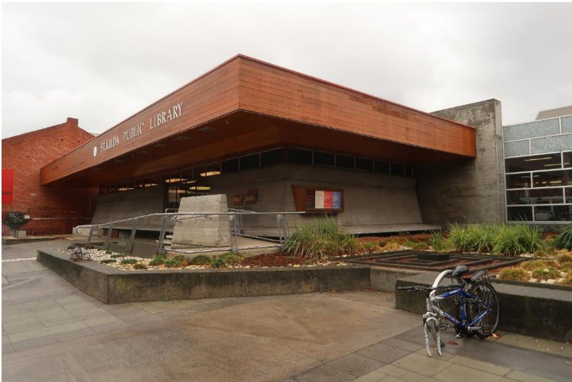
Figure 17 St Kilda Library, western (1973) sections of the Carlisle Street façade
