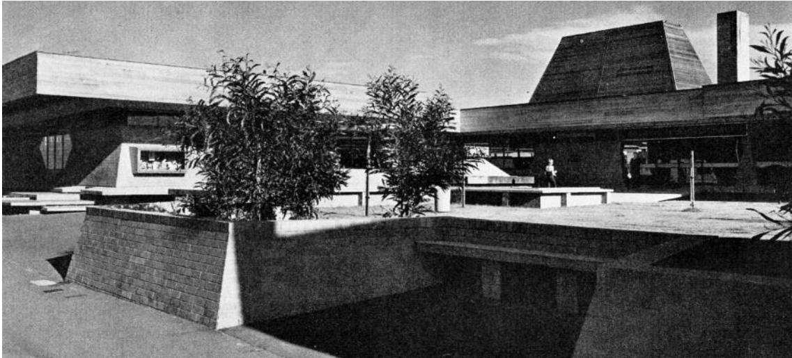
Figure 6 View of St Kilda Library from Carlisle Street, 1974 Source: Ian McKenzie, in Constructional Review , February 1974
