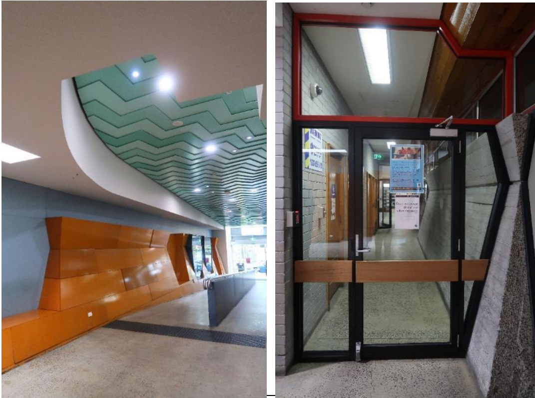
Figure 24 Disabled access ramp (left) and services corridor (right)
