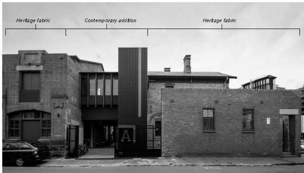
Photo 1: The adaptive re-use of the former Naval Drill Hall (left) and Port Melbourne Post Office (right) for the Albert Park College Environmental Arts Hub included this contemporary insertion linking the two buildings, as well as conservation works to the original buildings. Designed by Six Degrees architects, the complex was the recipient of a City of Port Phillip Design & Development Award in 2018.
