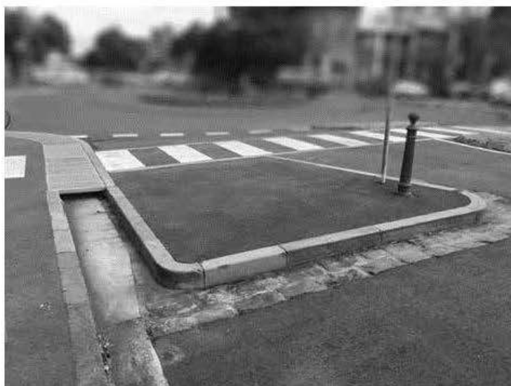
Photo 23. The installation of this new kerb outstand and associated pedestrian crossing in Bank Street, South Melbourne uses sympathetic materials and also ensures that the historic alignment and layout of the original kerb and channel remains evident.
