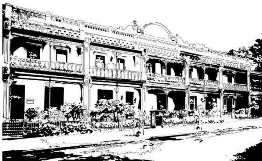
A typical symmetrical Victorian two-storey terrace row with distinctive vertical rhythm created by repetitive verandah bays and detailing.
