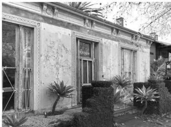
Photo 2. The removal of a c.1950s addition at the front of this house in Blessington Street, St Kilda revealed the original intact Victorian era façade. Outlines of the removed walls and some of the colour schemes, as well as the lower sections of the walls (now covered in vines) were left as evidence of this change.
