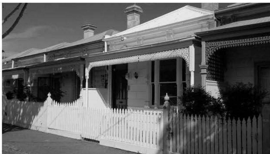
Photo 7. An example of a consistent residential streetscape
