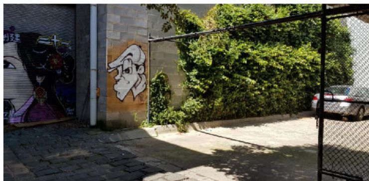
Looking at the access to the rear of the property at 119 Market Street from the Road
