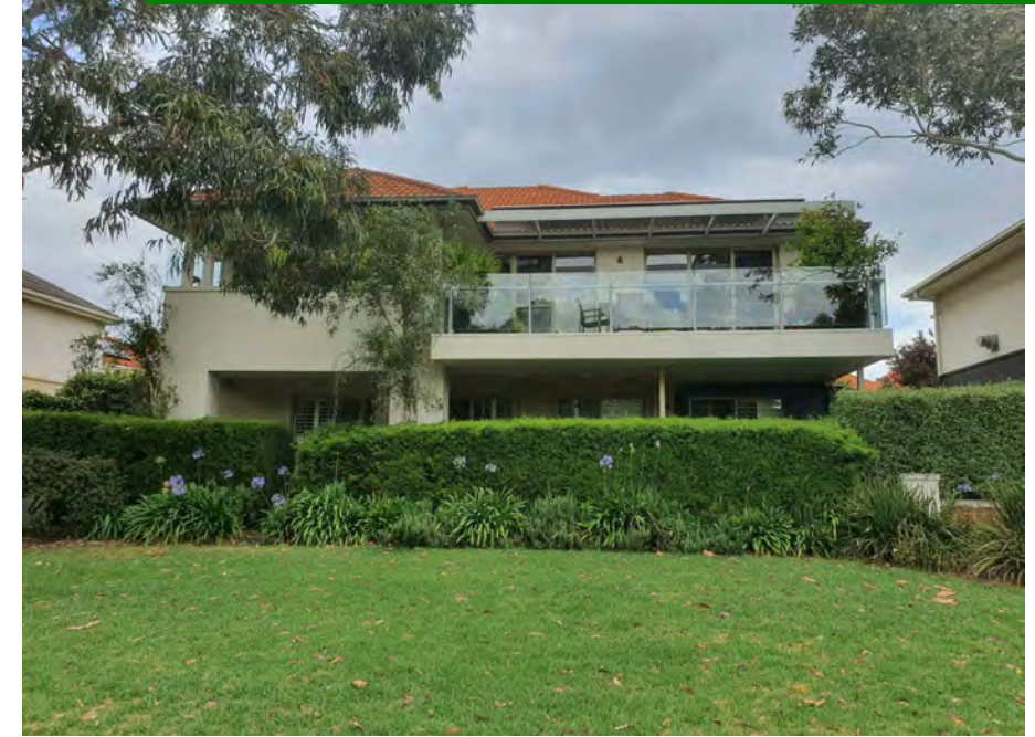
ADJACENT BUILDING FROM GARDEN CITY RESERVE
