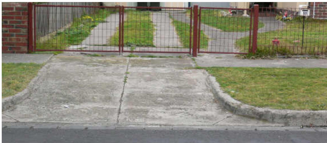
Figure 24: Driveway and pedestrian pathways as plain uncoloured concrete tracks, causing minimal use of hard pavings.
