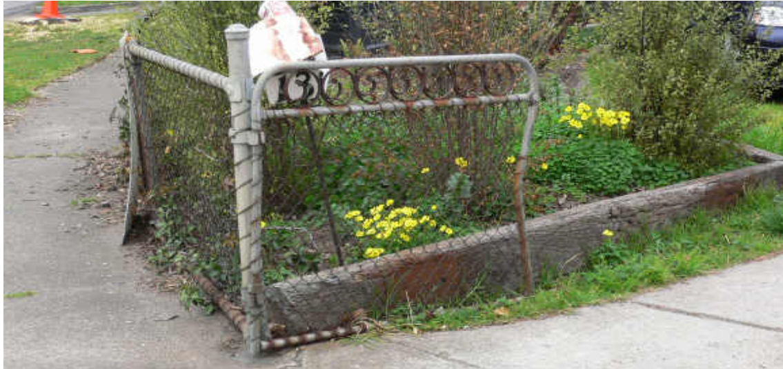
Figure 17: An early metal fence – Cyclone steel tube type (acceptable)
