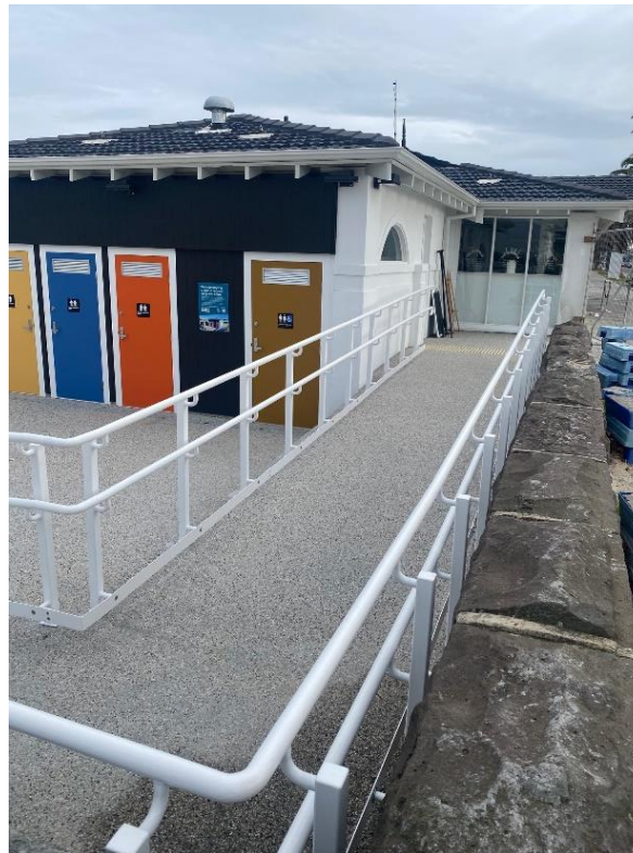
Upgraded public toilets at Sandbar
