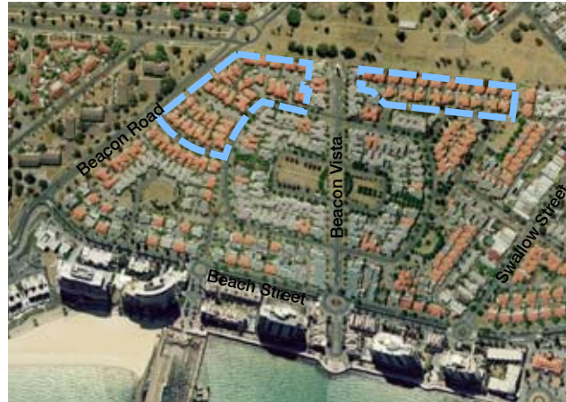
Figure 16: Aerial photograph of Precinct E
