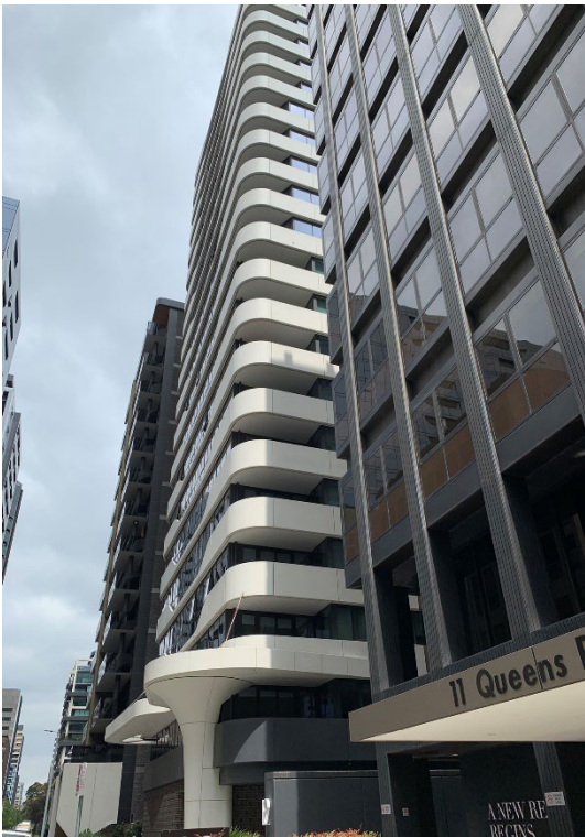
18. 12 Queens Road balcony to lane 02
