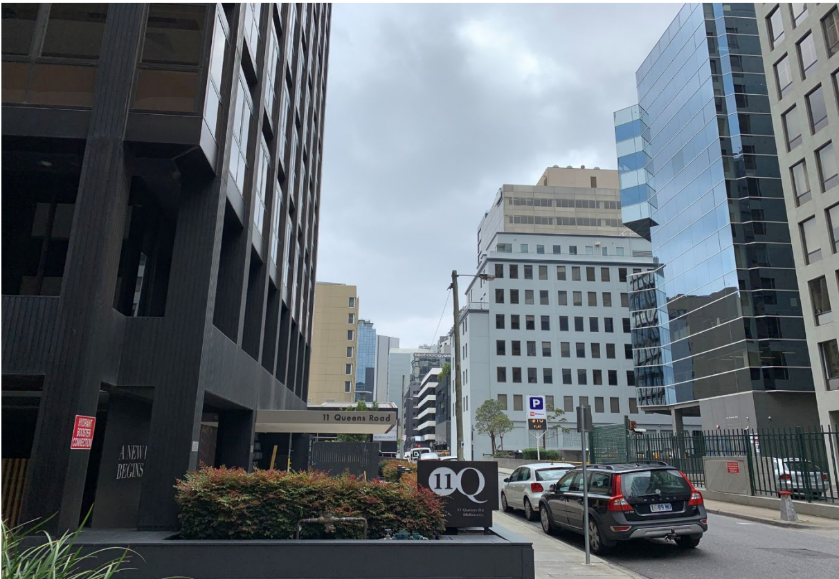
20. 11 Queens Road angle elevation to lane
