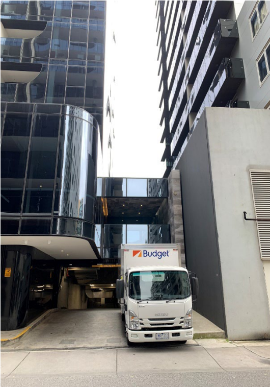
15. Side setbacks rear view between 450 & 452 from Queens Lane
