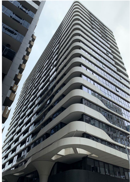
17. 12 Queens Road - Lane balcony view
