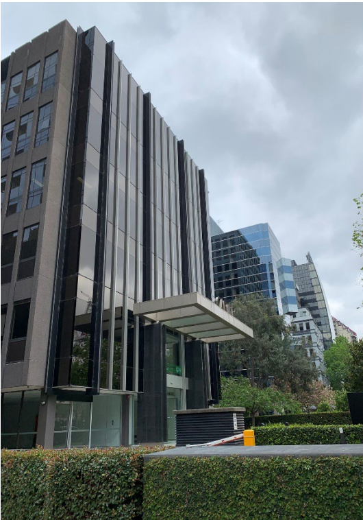
06. View from subject site southeast boundary looking north to 442 St Kilda Road
