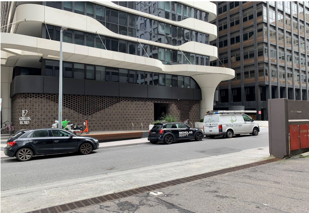
19. 12 Queens Lane ground floor rear elevation to Lane
