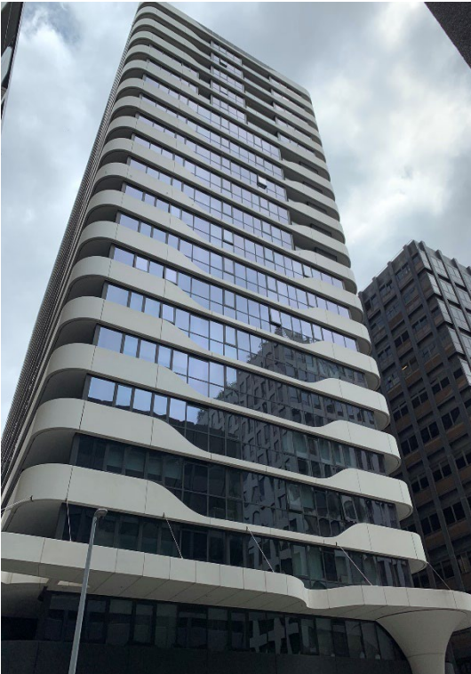
16. 12 Queens Road rear elevation to lane
