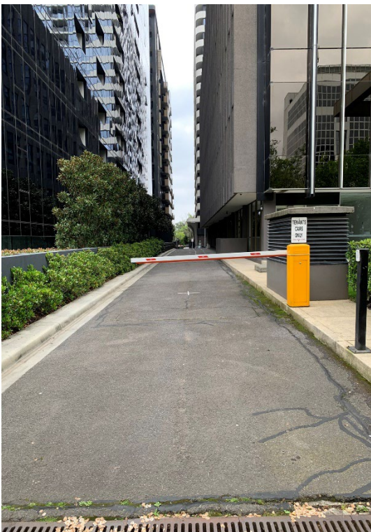
09. Subject site exiting accessway - view from St Kilda Road towards the rear Queens Lane
