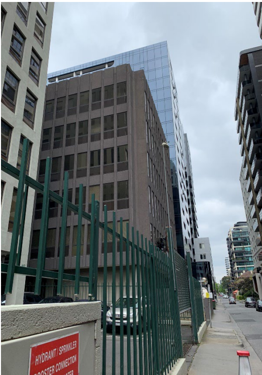
13. View to the subject sites' northern boundary with 442 St Kilda Road
