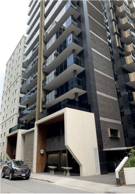
22. 14 Queens Road elevation to lane angle 01
