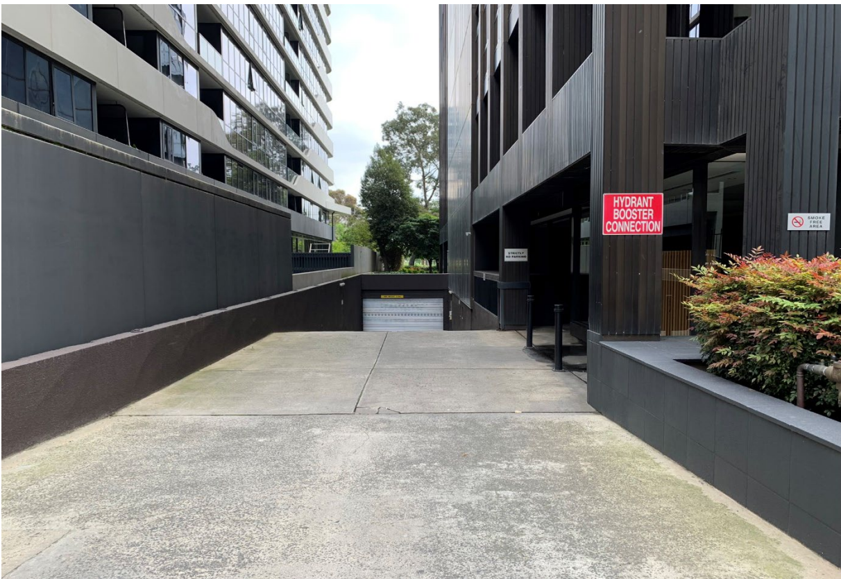
21. 11 Queens Road entrance to basement from lane
