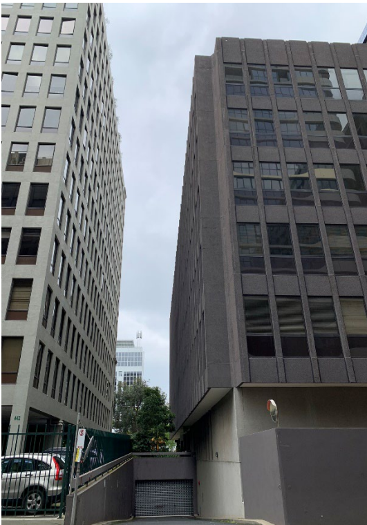
11. Long angle view to the rear of the subject site and side boundary to 442 St Kilda Road. Note the basement accessway.
