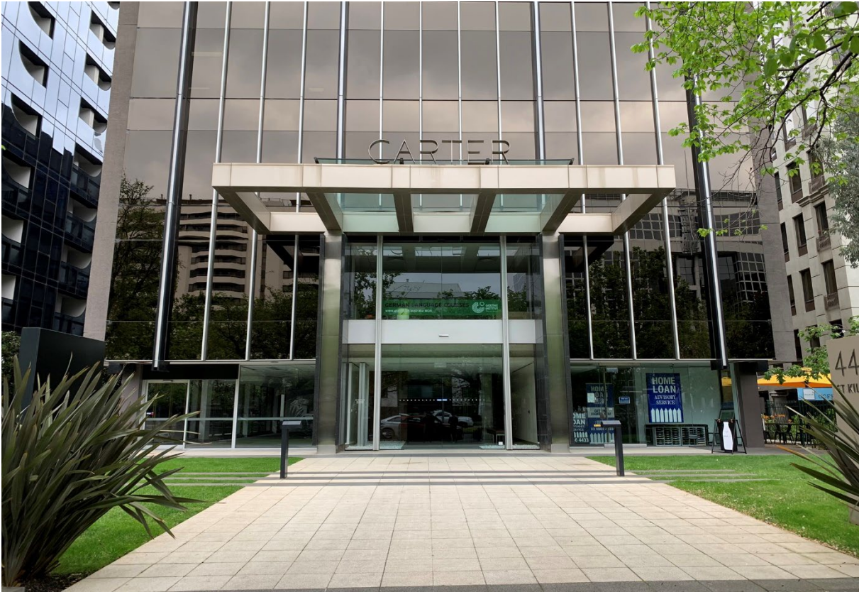
01. Subject site close up view to ground floor frontage
