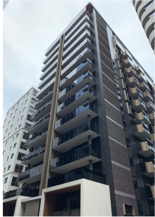
23. 14 Queens Road elevation to lane angle 02
