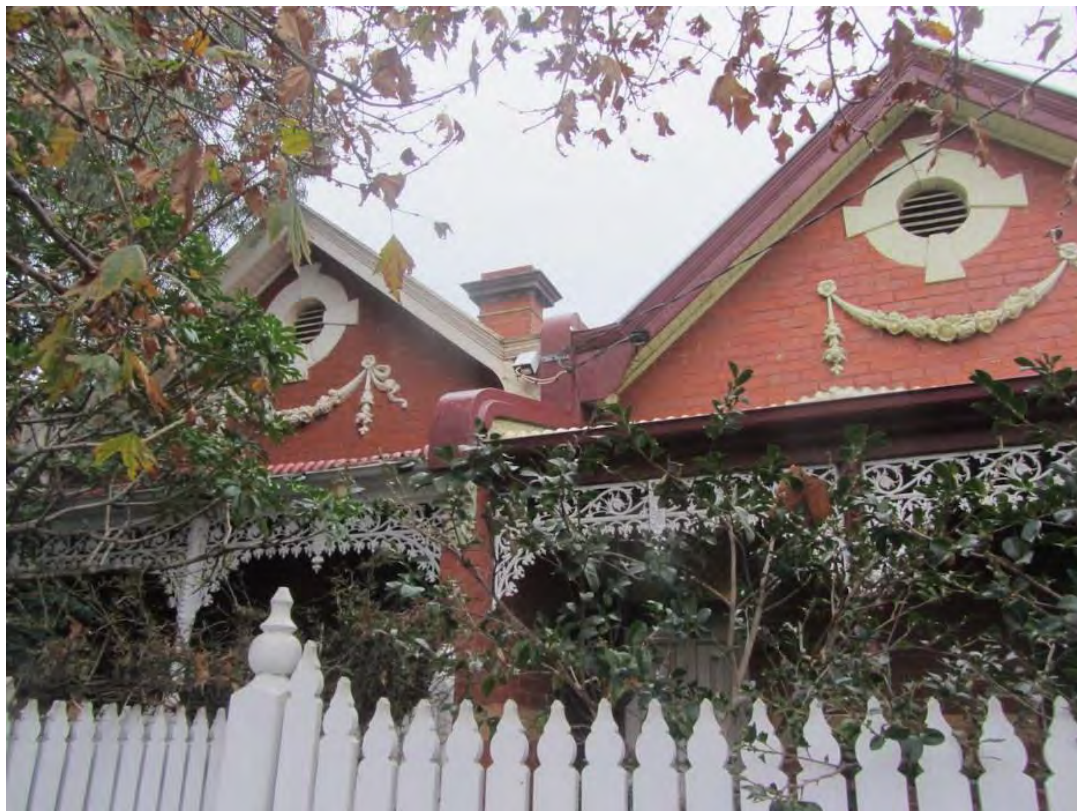
110-112 Barkly Street, showing the distinctive gable end detailing
