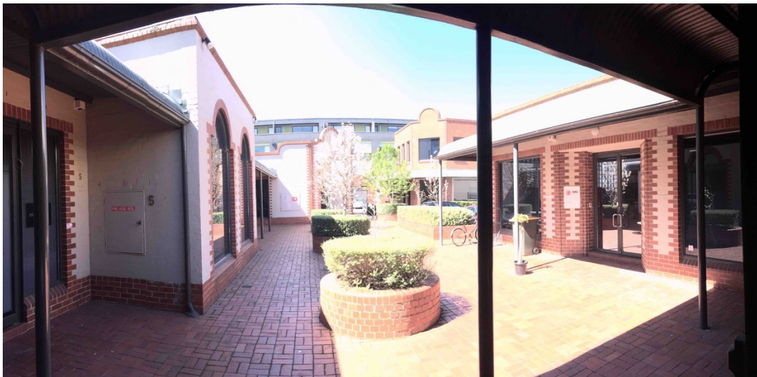
Figure 4 New development to the rear of the original laundry building
