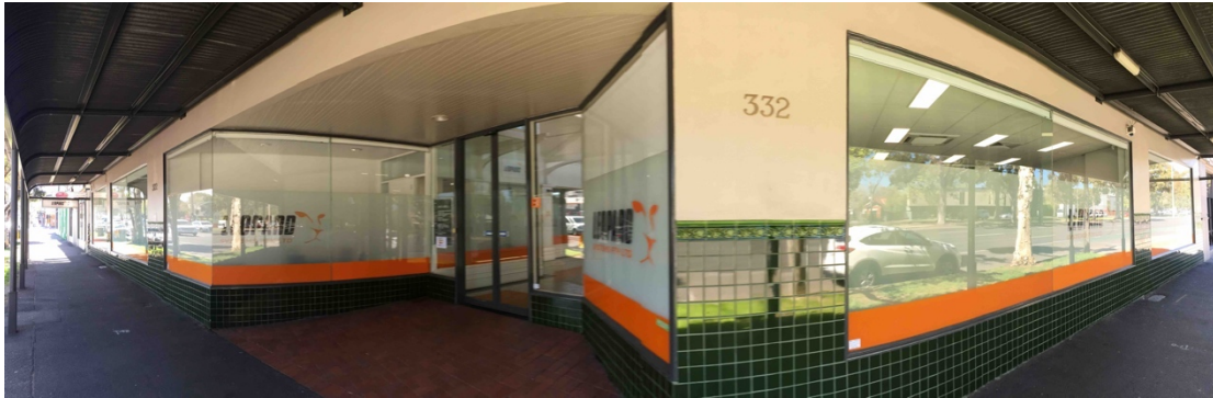
Figure 3 Shop fronts and veranda of the subject site that are wholly recent constructions
