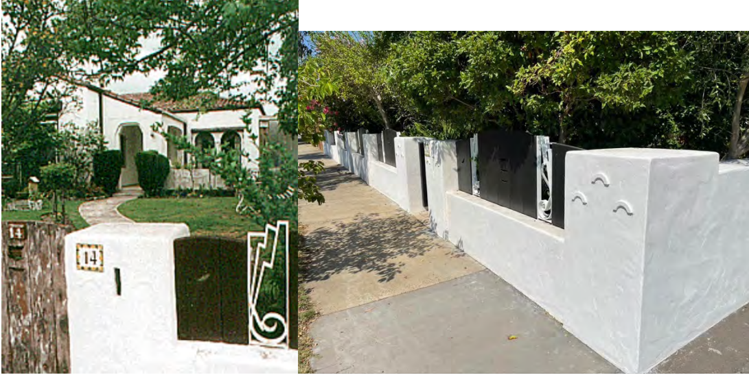
(Left) The house and fence c. 1998 (Source: Port Phillip Heritage Review) (Right) Front fence in 2022 following repair and conservation works
