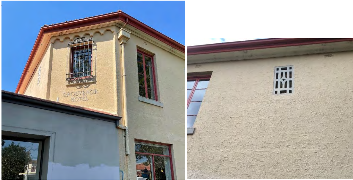
1. (Left) North-west splayed corner showing scalloped frieze, window with wrought iron screen and name plate (Right) Example of patterned inset wall screens
