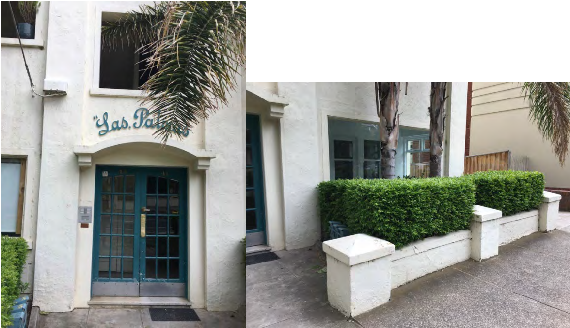
Las Palmas – entry and fence detail
