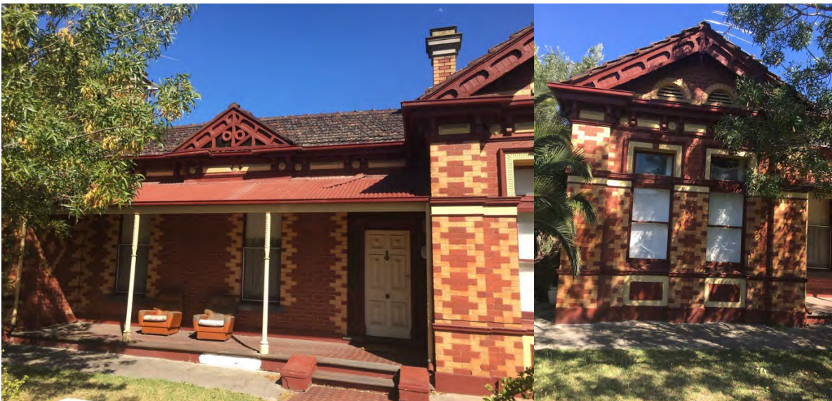
Verandah (also showing tiled path) and south gable of no. 33
