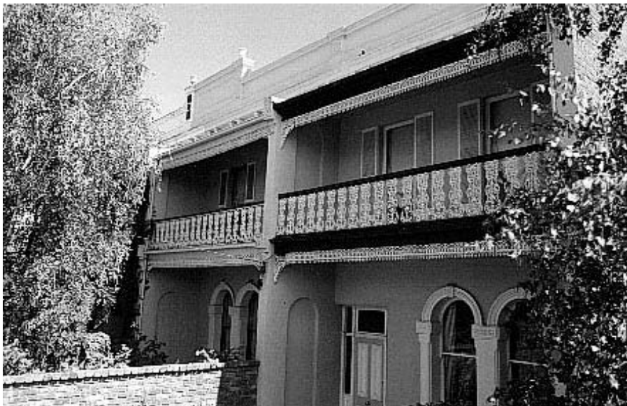
Figure 4 – The terrace at 113-119 Hotham Street showing the Romanesque window heads that are a characteristic of the houses in this precinct.
