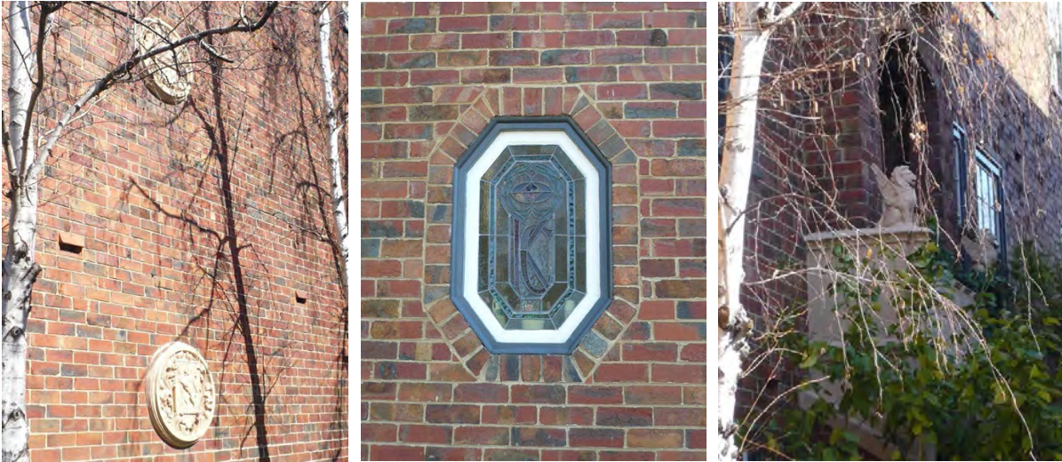
Building details from left: Medallions with heraldic symbols; octagonal leadlight glass window with pattern featuring an interlocked 'K' and 'C' in Gothic script; rendered balcony above entry to stairwell with Griffins in front of arched opening
