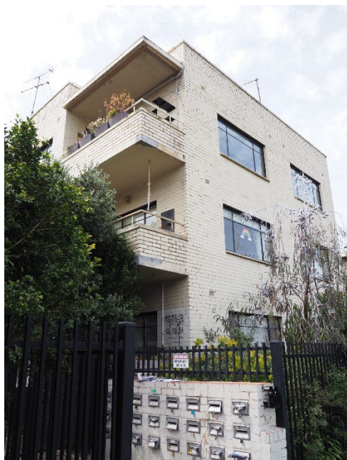
Figure 16 - Front elevation showing likely original brick letterbox wall
