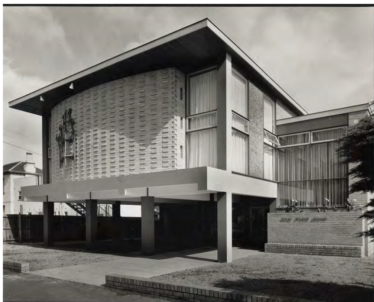
Figure 1: B'nai B'rith House (Hotham Street Reception Rooms), East St. Kilda 1960 (Source: State Library of Victoria, H2003.100/283)
