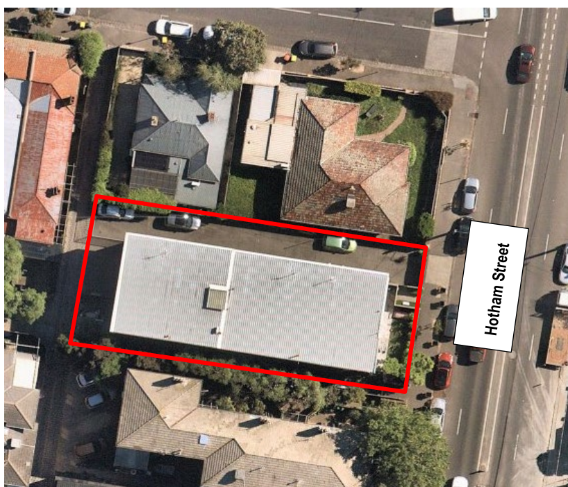
Figure 13 - Aerial showing extent of 169 Hotham Street, Balaclava. (Source: Nearmap, Oct 2021)
