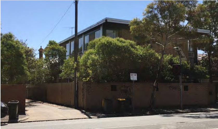
Side elevation in 2017 – note visible chimney of original house at rear
