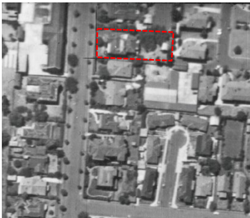
Figure 15 - 1945, showing former house at 8 Westbury Street (Source: Landata, Proj No 5, Run 18E, Frame 58014)
