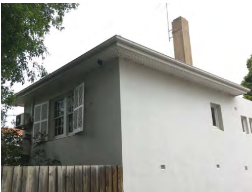
Below: former Chauffeur's quarters and garage at 4 Mitford Place.
