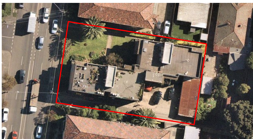
Figure 12 - Aerial photograph showing extent of 62 Hotham Street. (Source: Landata, October 2021)
