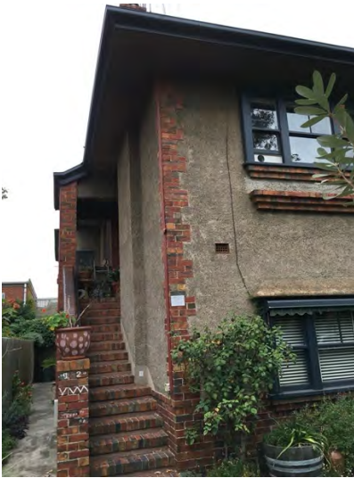
Detail of the east staircase
