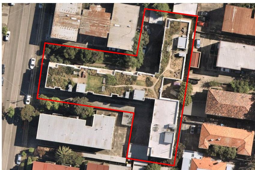
Figure 15 - Aerial photograph showing extent of 38 Westbury Street. (Source: Landata, October 2021)
