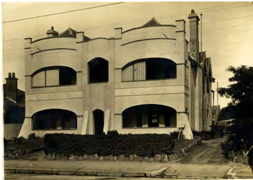
Figure 4: Queen's Court flats c. 1930 (Source: Port Phillip City Collection)
