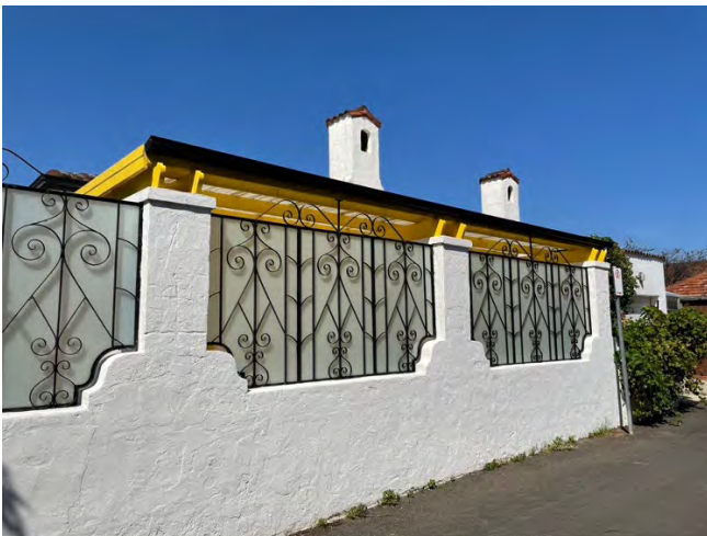
The original rendered piers of the side pergola and two of the 'dovecote' chimneys
