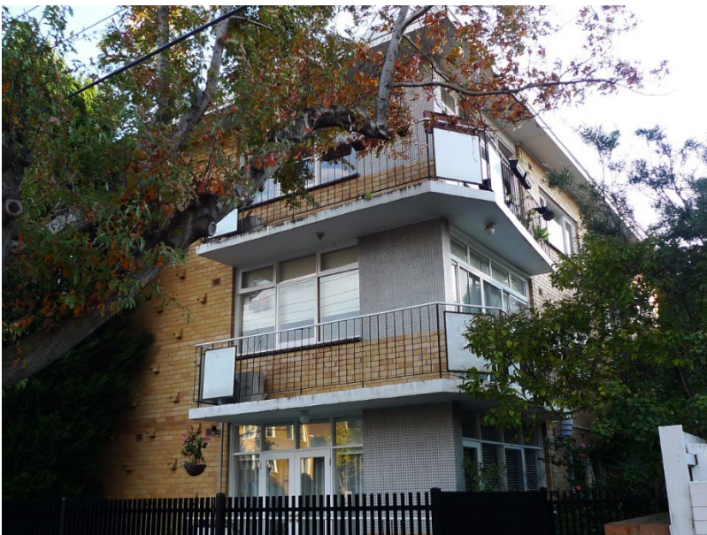
Figure 24 –North-east corner, showing splayed balconies
