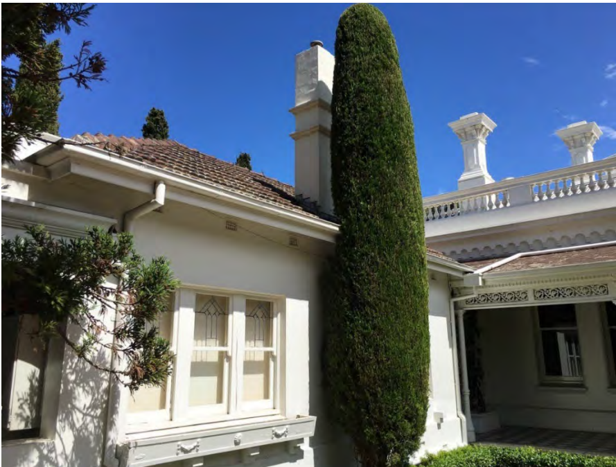
The 1935 addition at the south end of the east elevation
