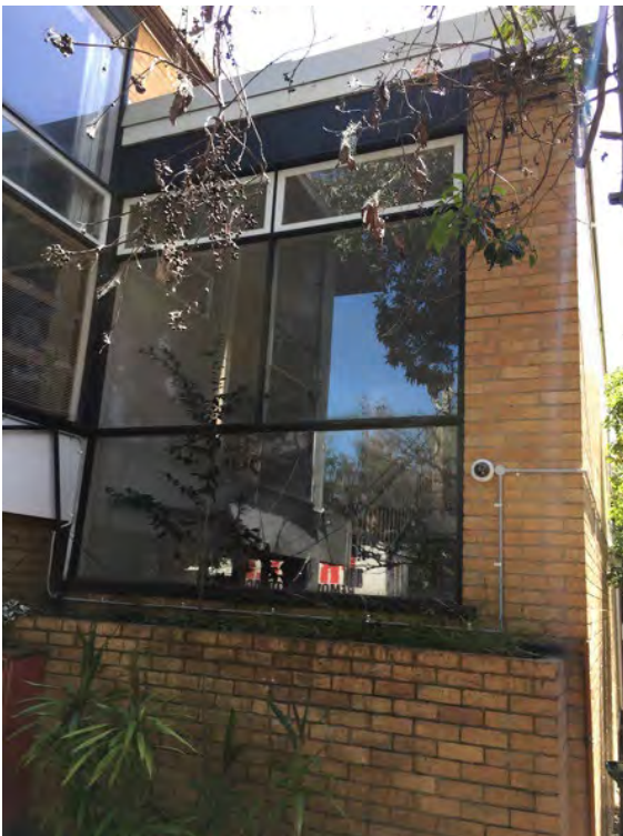
Stairwell of 1959 building in 2017 showing original window details
