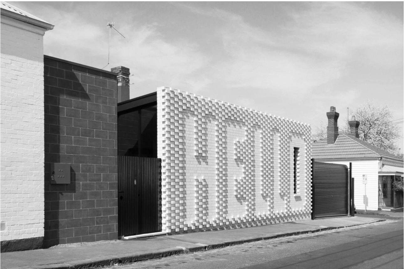
Photo 11. An extension featuring Hello wall by architect Fooi-Ling Khoo and graphic artist Rose Nolan. This design elevates a practical solution for privacy by creating "Hello" out of fine brickwork. It also showcases how contemporary design can contribute to the brick tradition of its 19th century heritage neighbours.
