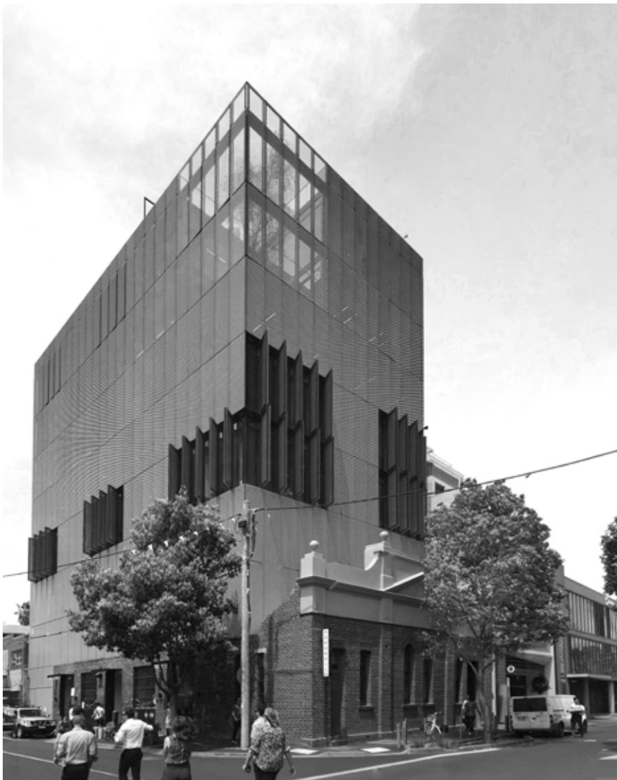
Photo 12. Lightweight material and simple details used for an office addition above a Federation era factory of local significance in Cremorne Street, Richmond.
