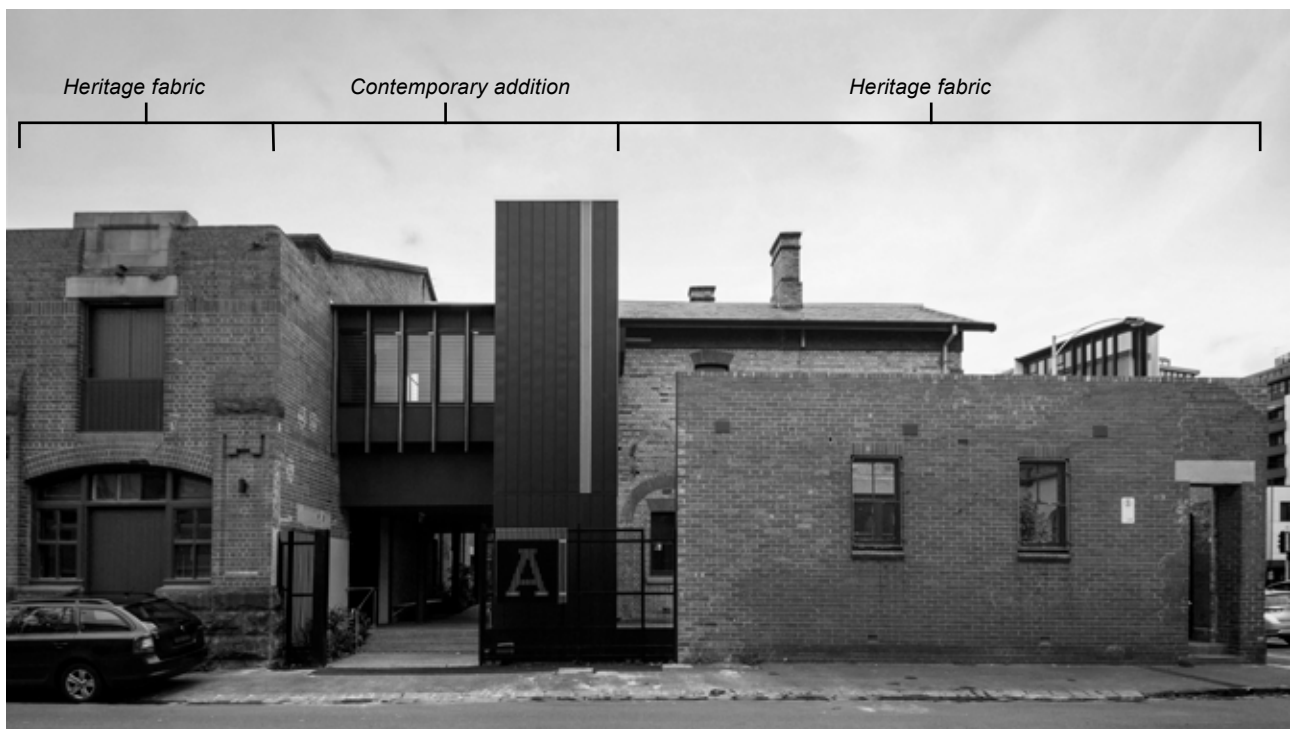
Photo 1: The adaptive re-use of the former Naval Drill Hall (left) and Port Melbourne Post Office (right) for the Albert Park College Environmental Arts Hub included this contemporary insertion linking the two buildings, as well as conservation works to the original buildings. Designed by Six Degrees architects, the complex was the recipient of a City of Port Phillip Design & Development Award in 2018.
