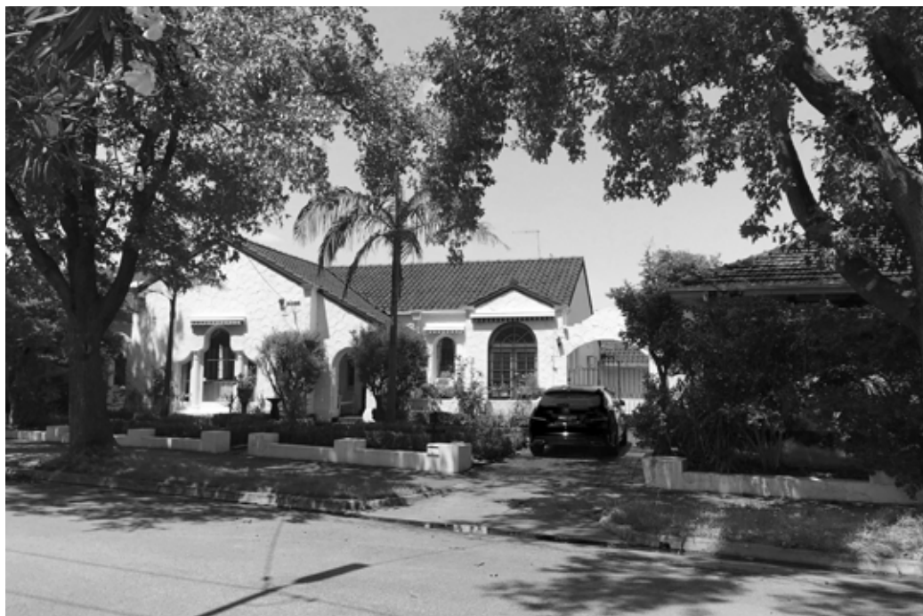
Photo 17. The original driveway and crossover, Los Angeles Court, Ripponlea
