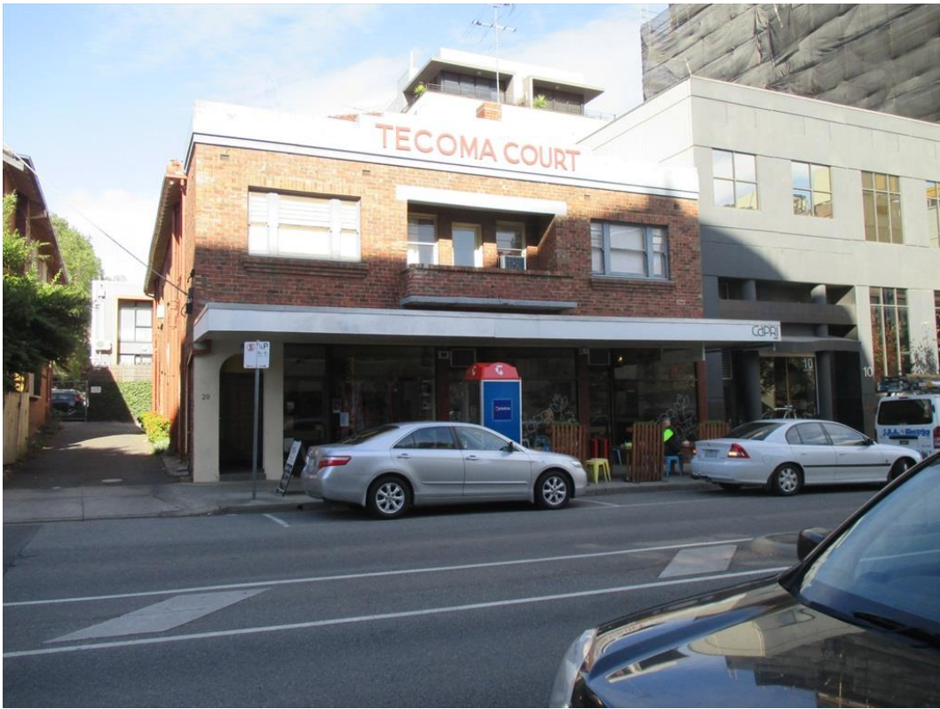
Figure 8 Wellington Street elevation of Tecoma Court, 16-20A Wellington Street.
