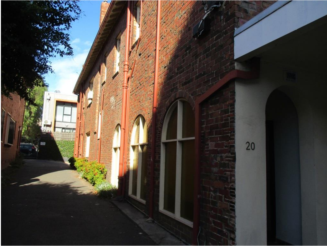
Figure 10 East elevation of 16-20A Wellington Street.
