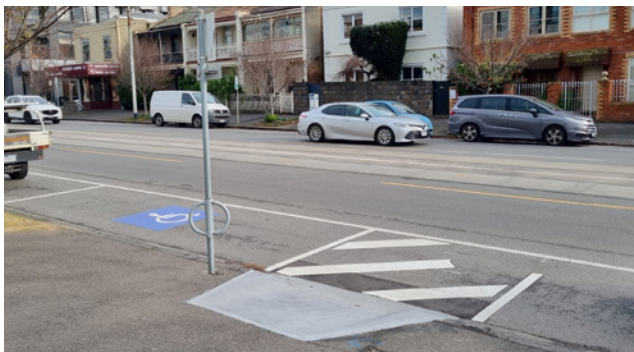
Park Street upgraded parking space.
