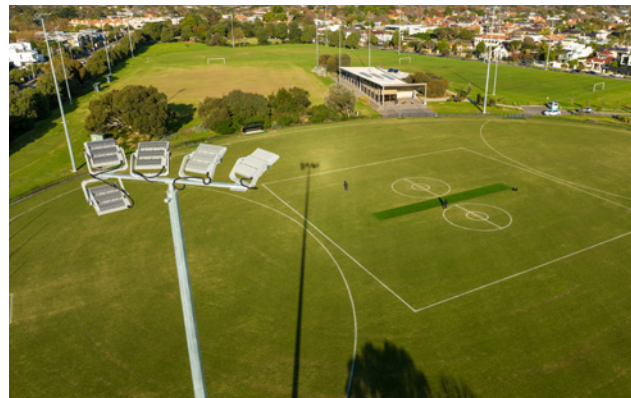
New lighting upgrade at Elwood Park.
