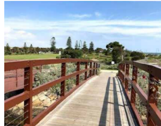
Moran Reserve Bridge, Elwood.
