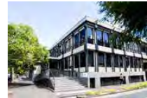
Late 20 century office building
