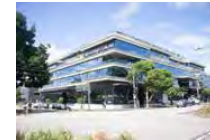
Large format commercial building
