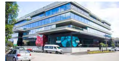
Four Storey Street Walls
