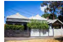
Victorian worker's cottages
