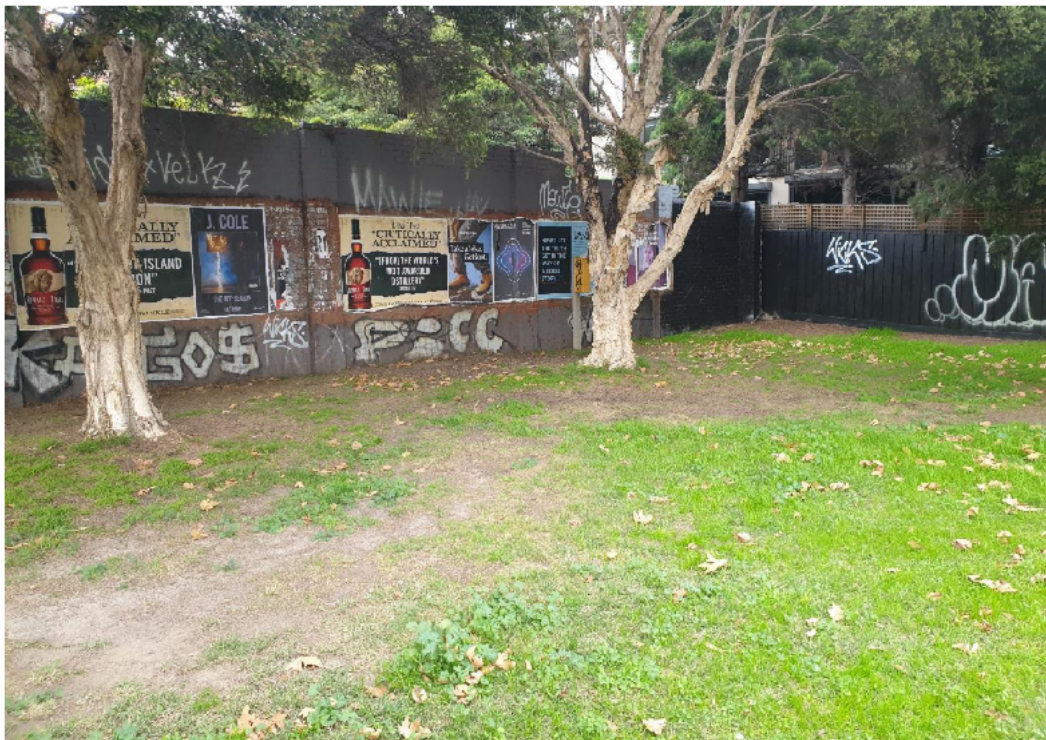
Photograph 2: View facing the southern portion of site. The brick fence along the southern boundary is a remaining wall from a demolished building.
