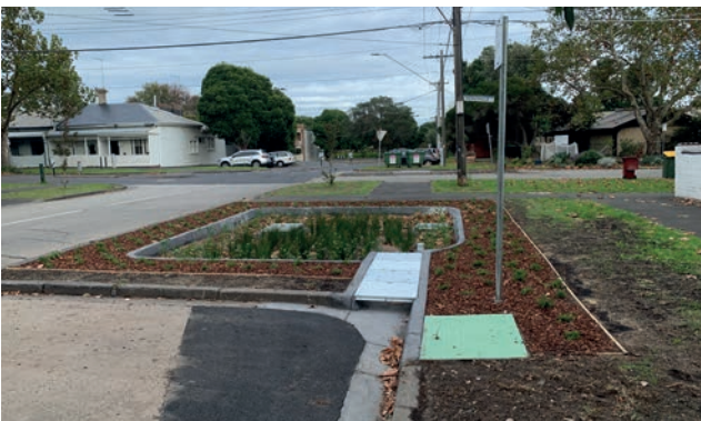
Raingarden at the intersection of Coventry and Montague streets in South Melbourne.
