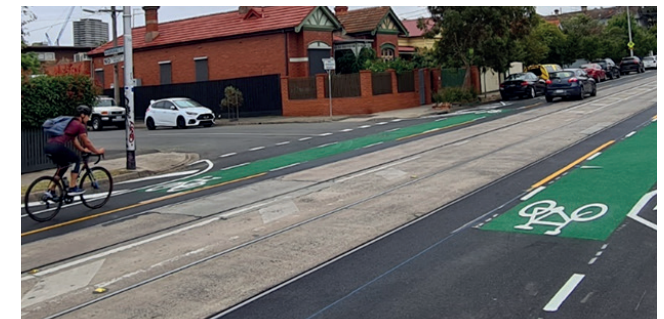
Chapel Street with green pavement marking with bike lane and painted islands.
