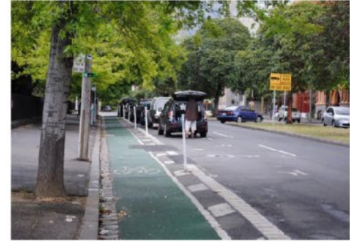
Example of temporary road arrangement at Albert Street, East Melbourne. Photos: Lorenza Casini
