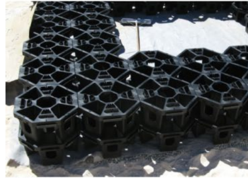
Structural Soil System
