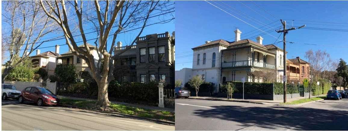
Figure 6.10 Error! No text of specified style in document.–11 – Italianate villas at 3 & 5 Crimea Street (left) and 100 & 98 Wellington Street (right)
