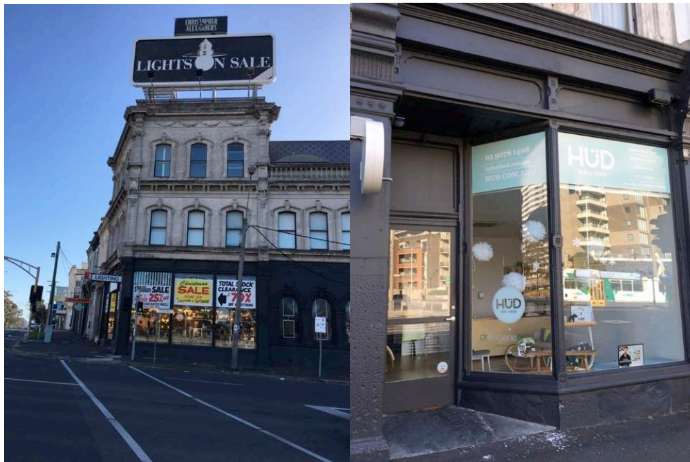
Figure 6.10 Error! No text of specified style in document.–19 – 140-146 St Kilda Road, with one of the original shopfronts at right
