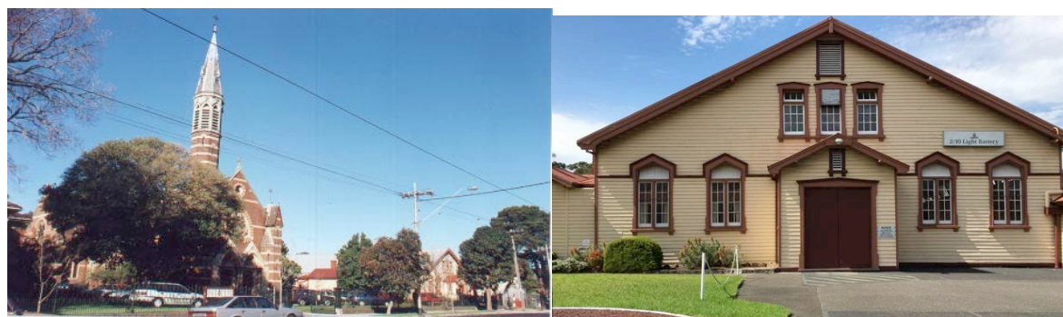
Figure Error! No text of specified style in document.–8 – St. George's Uniting (former Presbyterian) church of 1877-80 and the former St. Kilda Orderly Room dominate the Chapel Street hill
