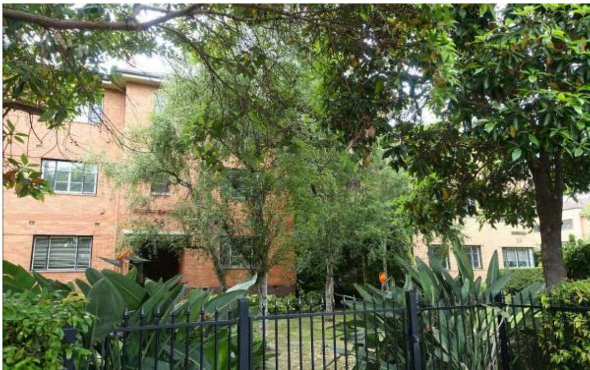
Figure 3 Streetscape photograph of part 58-60 Queens Road, Melbourne (Source: Ms Schmeder’s expert report, page 47)
