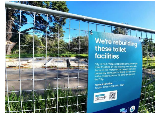
Reconstruction commenced on the Alma Park Pavilion in August.
