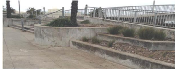
St Kilda Esplanade footbridge 'before'
