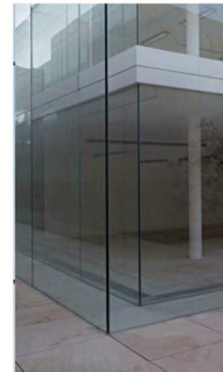
GLA01 Clear Glazing Total glass/frame system to achieve thermal performance as required by ESD and Facade consultants Max reflectivity 20%
