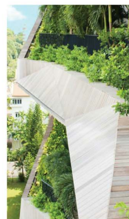
CONC05 GRC planter boxes with travertine finish. GRC cladding over mild steel sub framing to be integrated into planter boxes
