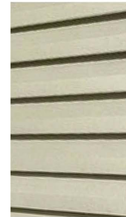
MET03 Pre-finished anodized 3mm thick solid aluminium louvre. Matte finish. Colour: To match MET01
