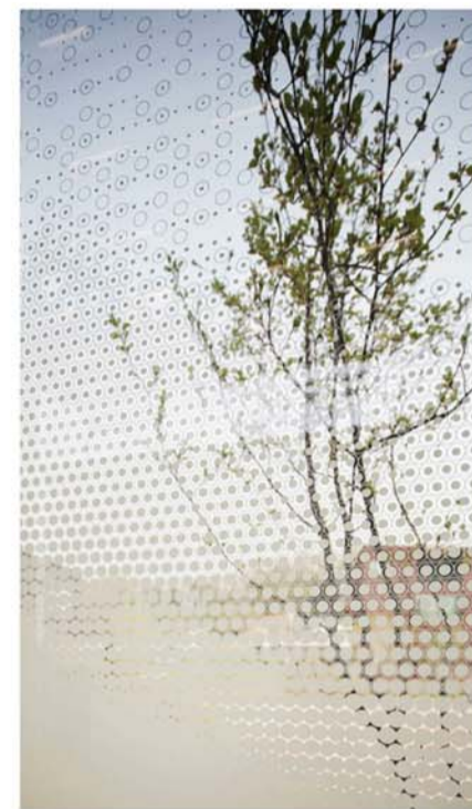
GLA03 Glazing with custom frit Total glass/frame system to achieve thermal performance as required by ESD and Facade consultants Max reflectivity 20%. Glazing to have custom ceramic frit.
