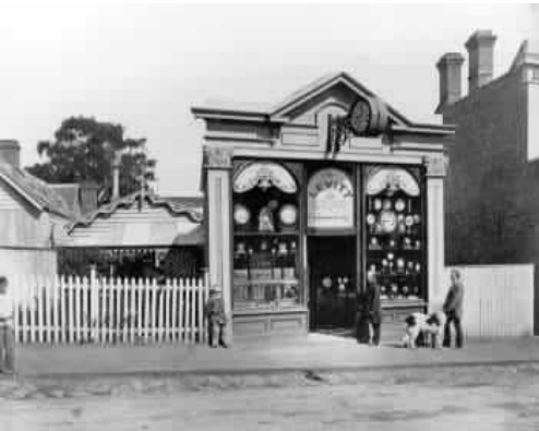
Former western side of High Street (St Kilda Road)
