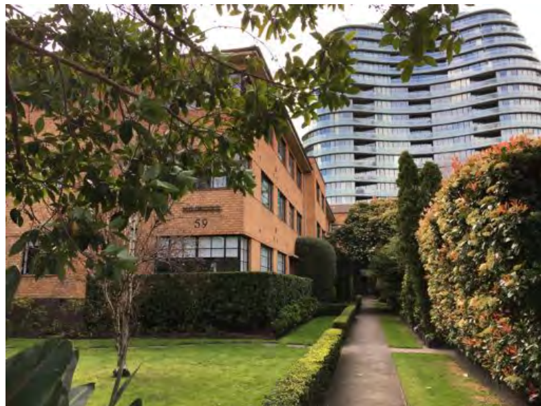
Kinross, 59 Queens Road, is situated towards the centre of the site.
