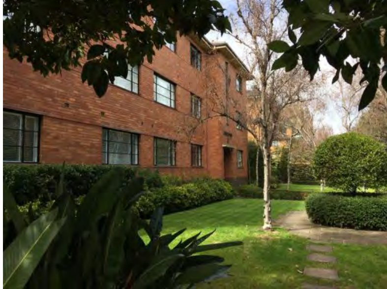
Glen Eagles, 58 Queens Road, west elevation facing Queens Road. The other two blocks in this complex, Kinross and Kinfauns, are partially visible at right.
