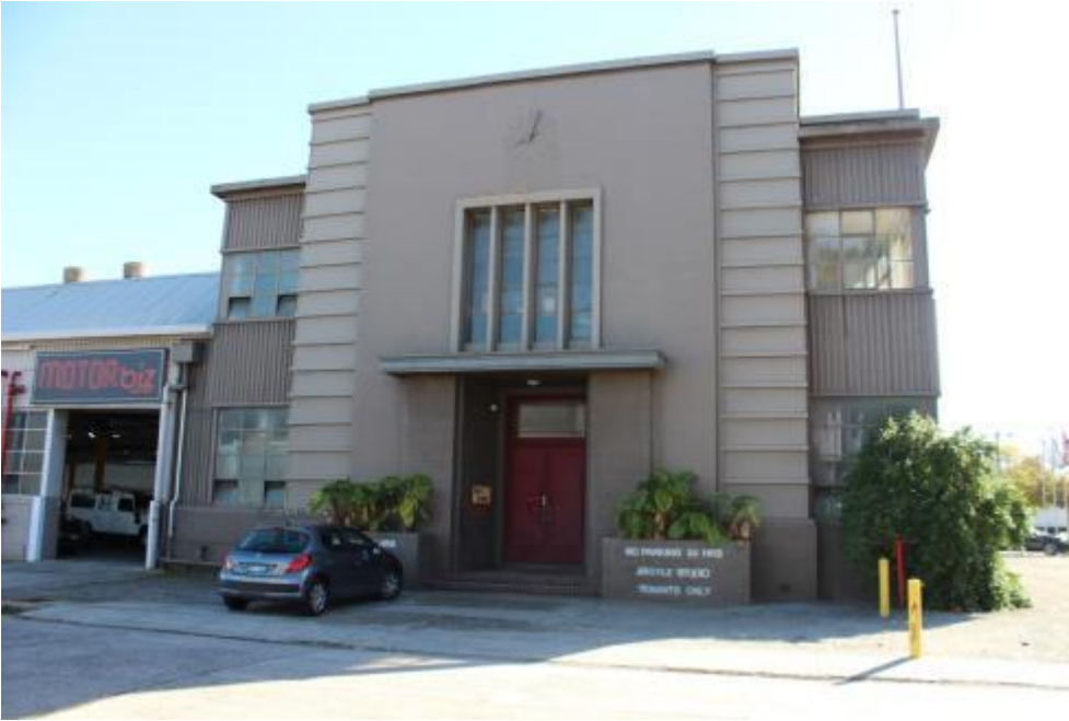
Figure 64: Main entrance, south elevation. Note clock above first floor windows
