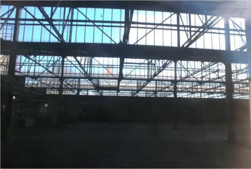
Figure 70: Rooflights of western assembly building (west of Smith St)
