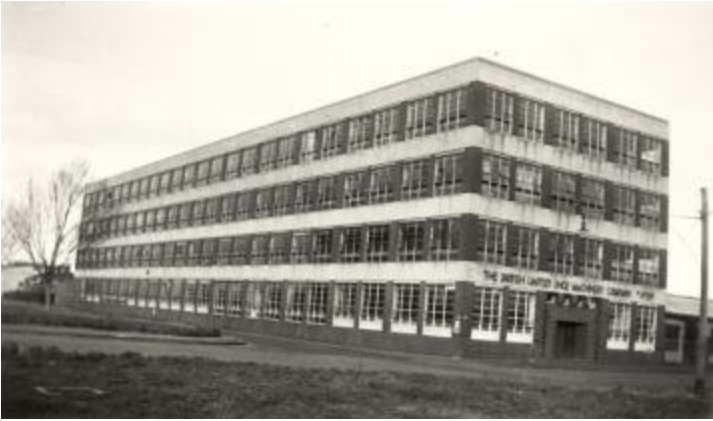
Figure 11: British United Shoe Machinery Company, 1948, Alexandra Parade, Fitzroy. Fitzroy Library ID: 15232
