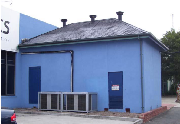
Figure 53: Substation Hyde Street Yarraville designed by Joseph Plottel, with simple pavilion design. 71
