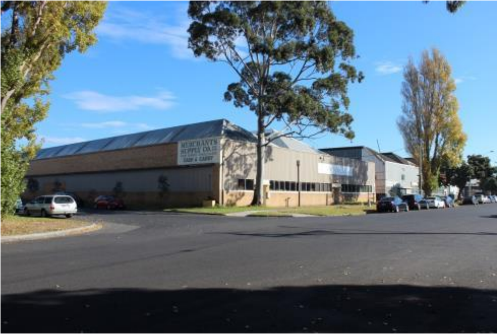
Figure 68: Assembly buildings west of Smith Street looking north west
