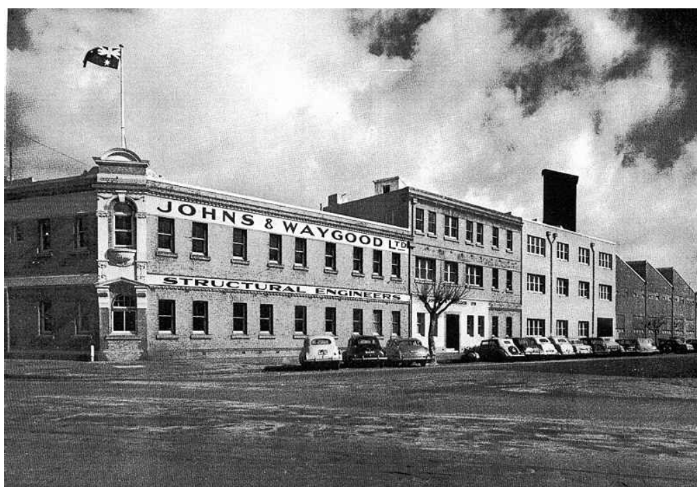
Photo: original Johns & Waygood premises, corner Cecil Street & City Road.
