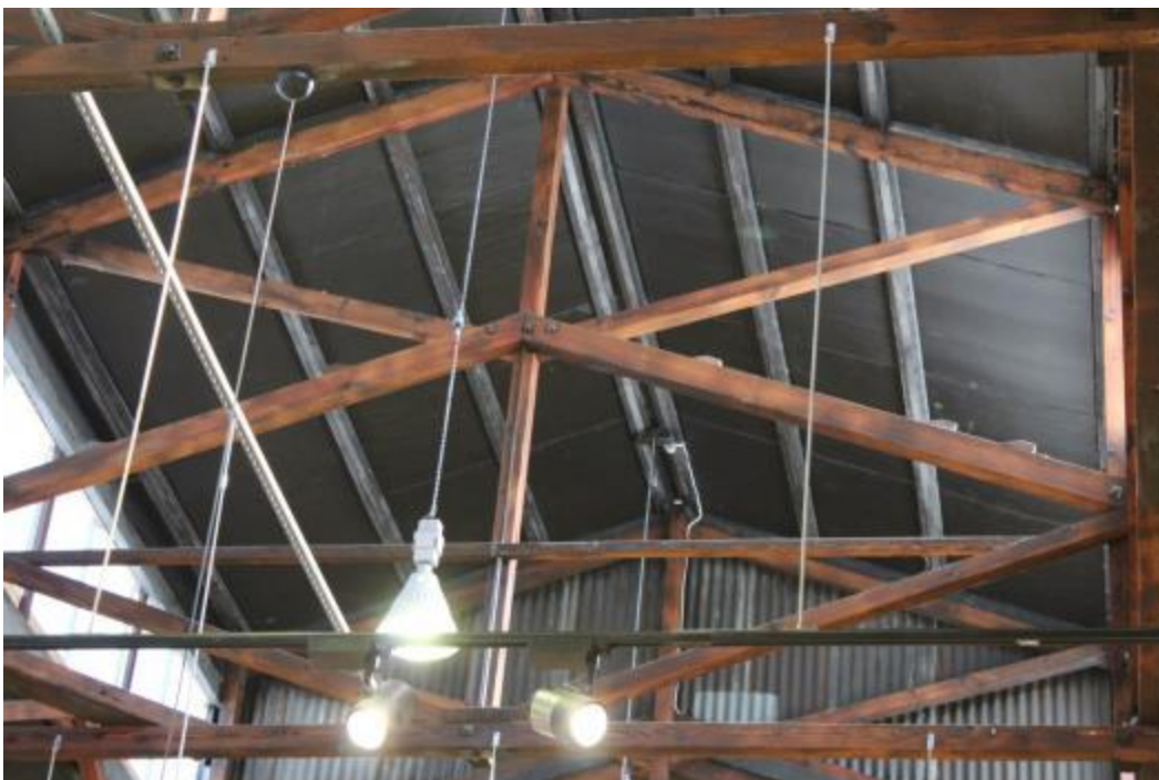
Figure 23: Interior roof truss detail
