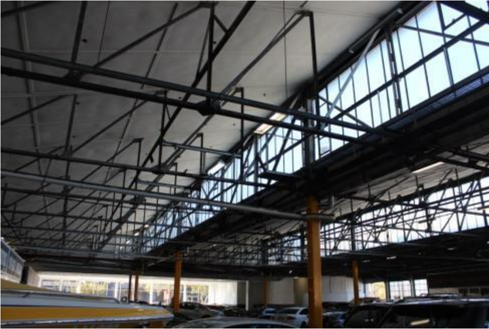
Figure 72: Interior of main assembly building looking west
