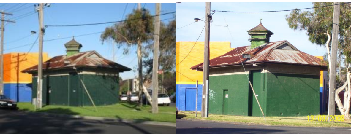
Figure 47: Electricity Substation from Johnston Street looking south west
