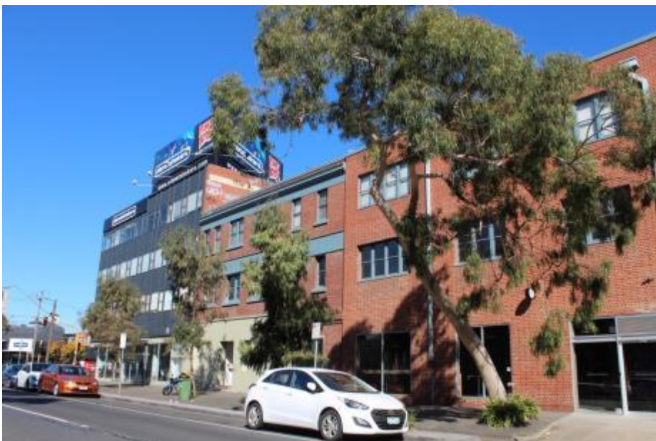
Figure 17: Elevation along Cecil Street looking north
