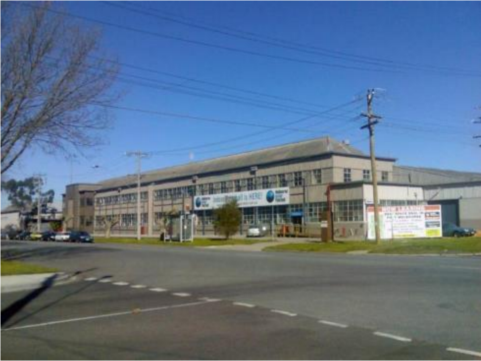
Figure 62: Rootes Main office buildings on Salmon St.
