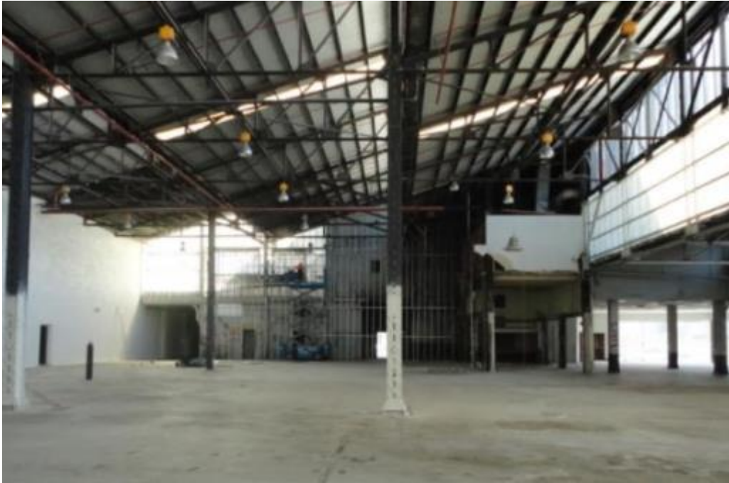
Figure 22: Main erection shop looking towards Cecil Street.
