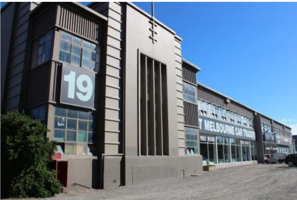
Figure 63: East elevation of office block with flagpole
