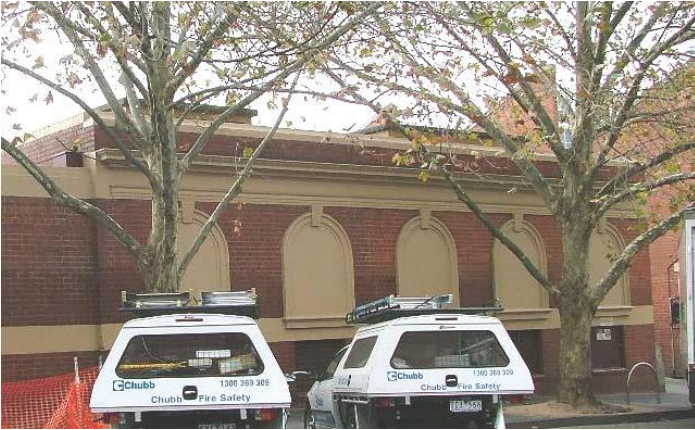
Figure 50: Substation, Substation, 70 to 74 Therry Street Melbourne, c.1928, a somewhat different Melbourne example with simple exposed brickwork, heavy moulded cornice above false arch opening.
