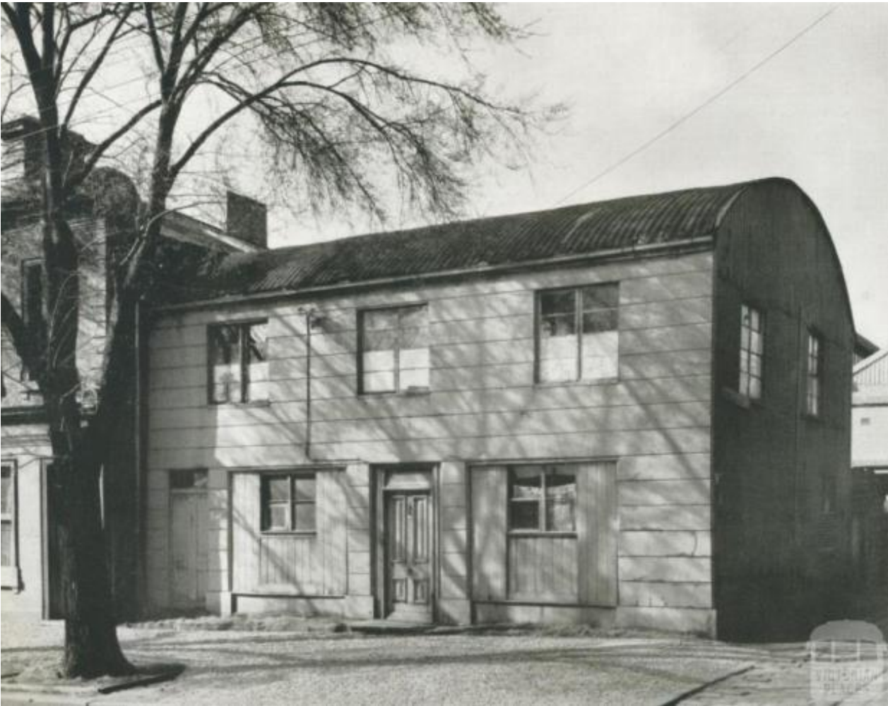
Figure 32: Pre-fabricated Iron House, 1956. This is presumed to be imported by Peter Johns, Johns & Waygood Limited (1856-1956) John Young Collection http://www.victorianplaces.com.au/node/64315
