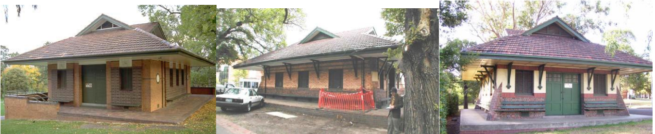
Figure 49: MCC pavilion substations: Clarendon Street, Fitzroy Gardens; Substation 10, Opposite 50 Jolimont Street, Jolimont 1938; Royal Park at corner of Royal Parade and the Avenue, Parkville.
