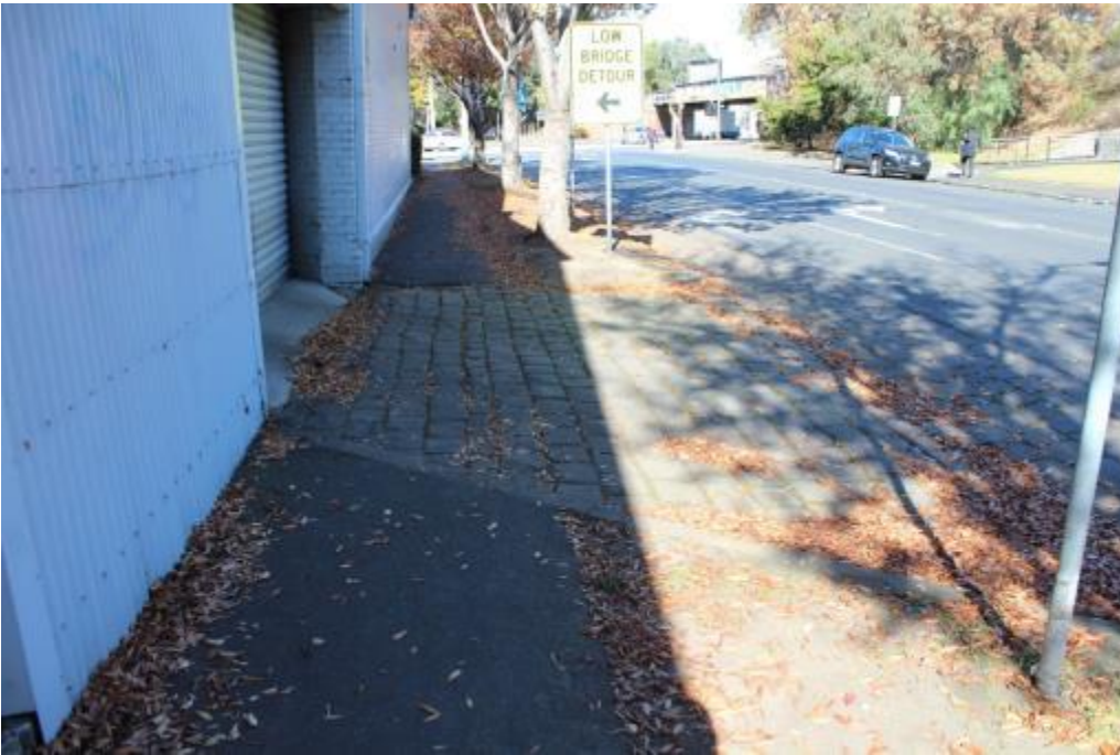
Figure 30: Bluestone cobbled vehicle entry and crossover at Whiteman Street
