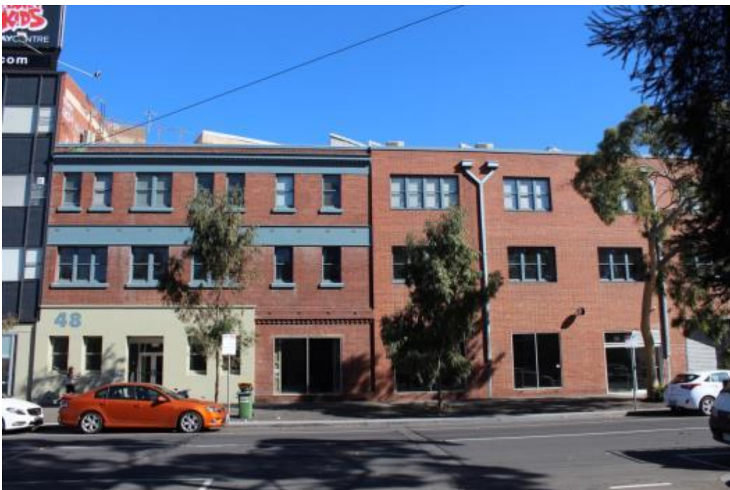
Figure 19: C1910 general store and c1920 machine shop along Cecil St.
