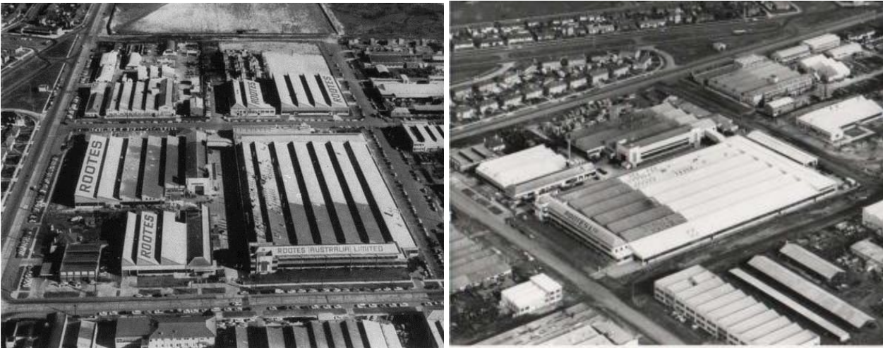
Figure 80: Rootes Factory looking west, Williamstown Road on the left 108 and south west. 109
