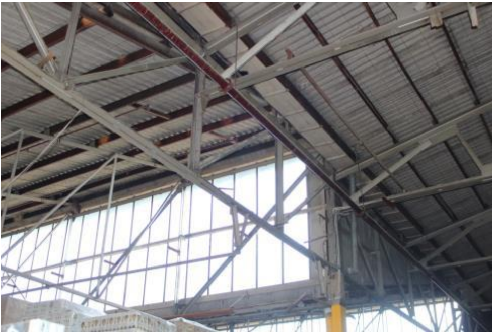
Figure 71: Roof trusses of main assembly buildings
