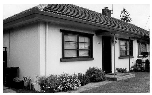
Figure 25. The original details of a concrete dwelling. Note the splayed eaves verge and splayed gutter, the eaves boxing, the partially concealed downpipe and the sliding timber windows with horizontal glazing bars set directly in the projecting concrete architrave in which the tracks are located.
