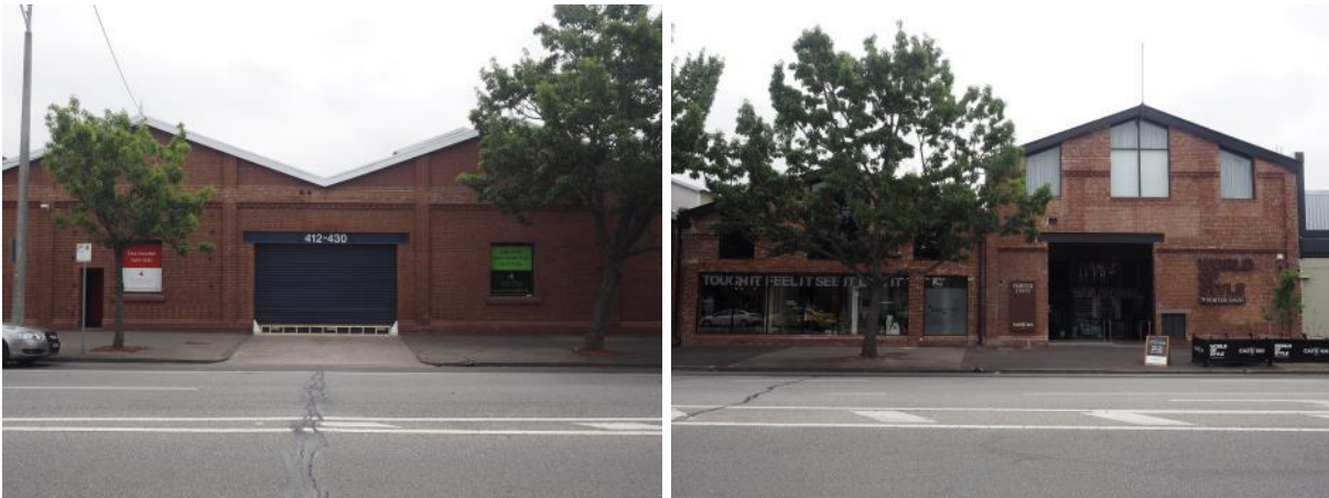
Figure 3 – Facades of 408 – 430 City Road (numbered right to left)
