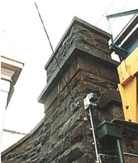
Carlisle Street bridge pier detail
