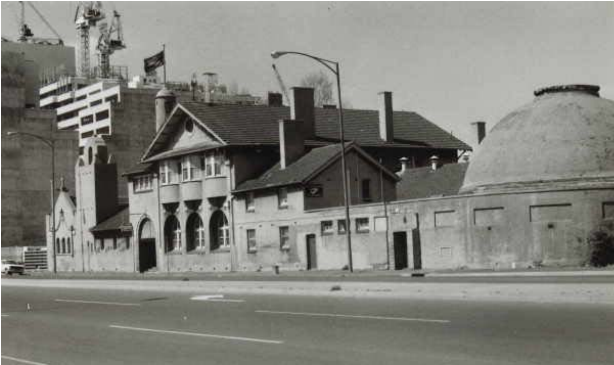
Figure 2 The former Anglican Missions to Seamen, now the Mission to Seafarers (1917), Flinders Street extension, Docklands, photographed in 1981. Source: John T Collins collection, State Library of Victoria.
