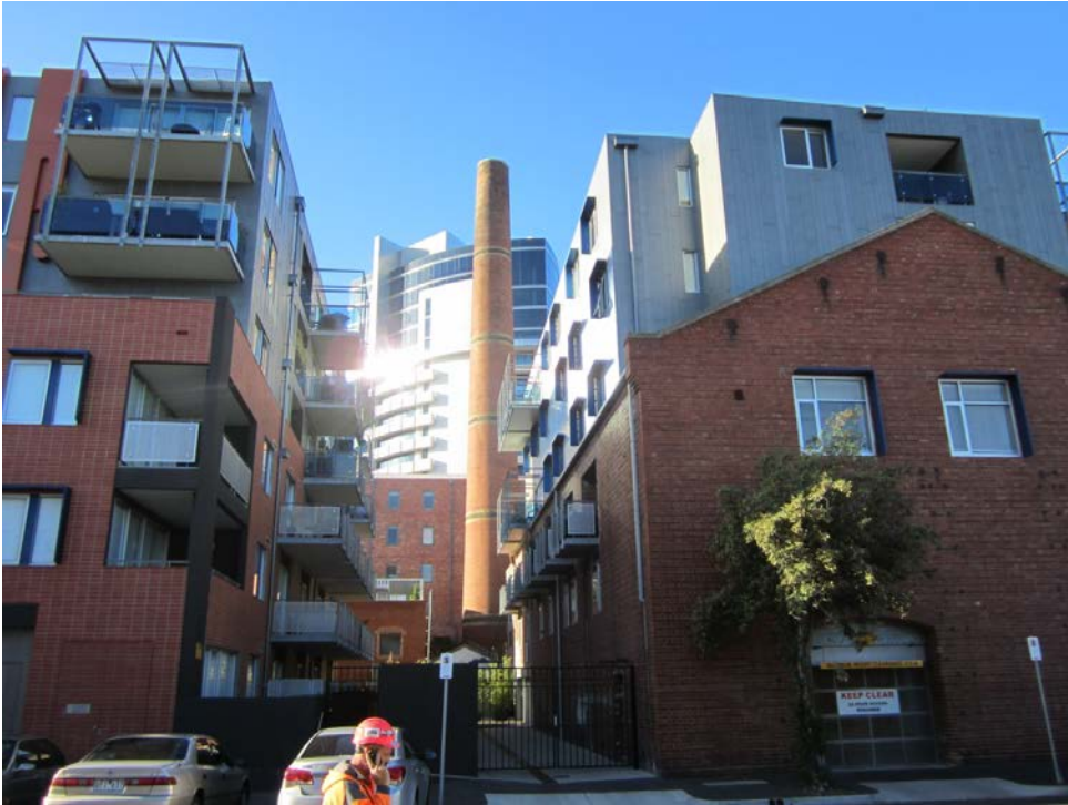
Figure 5 50 Dow Street shown at right, looking east, showing the 2009 residential conversion of former factory building. The adjoining building at left – 52 Dow Street – is not contained within the heritage overlay.
