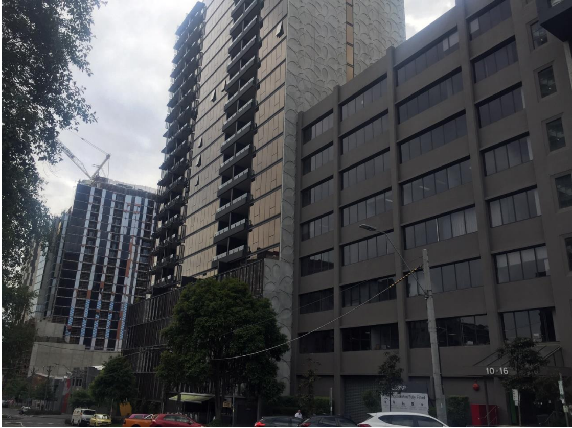
Existing built form opposite the subject site
