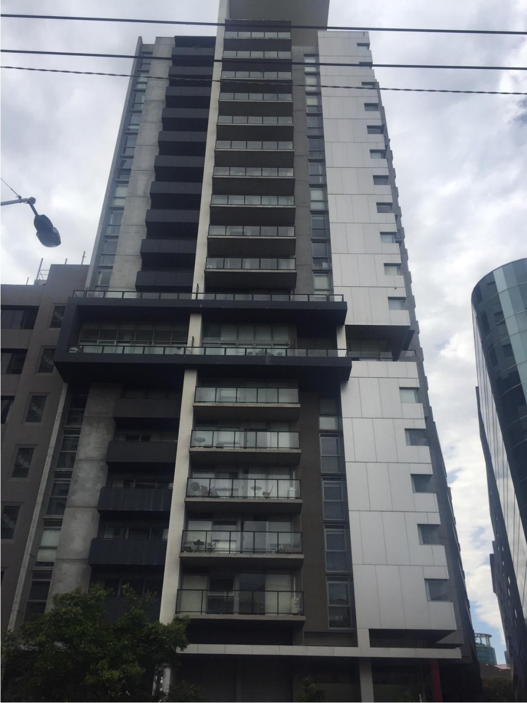
Example of built form to the rear of the subject site
