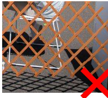
Figure 13: Flimsy materials like lattice should not be used in parklets
