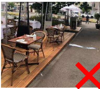
Figure 23: Platform is not flush with surround footpaths
