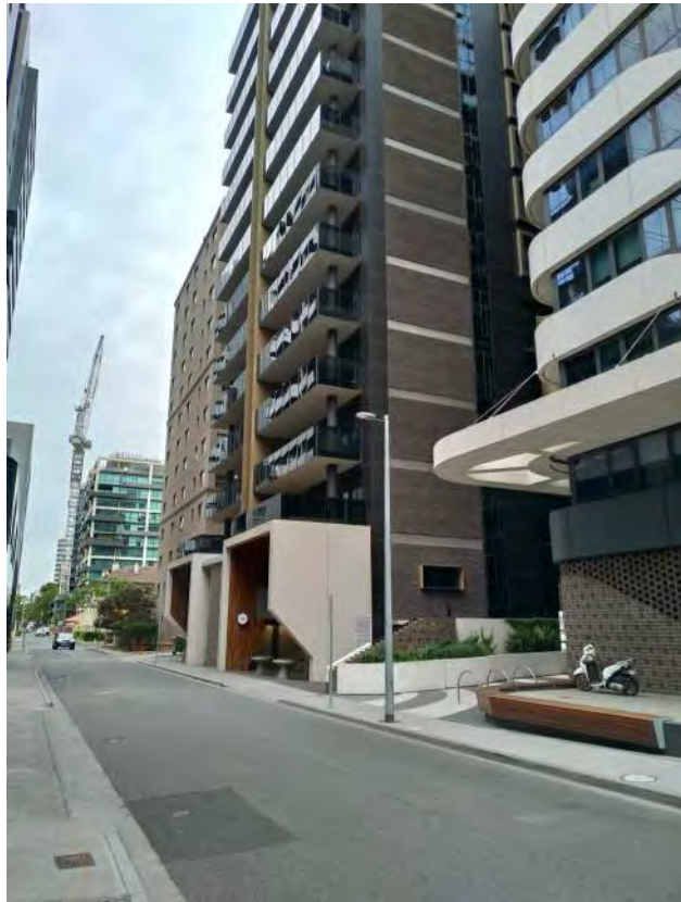
10 14 QUEENS ROAD AND 12 QUEENS ROAD.
