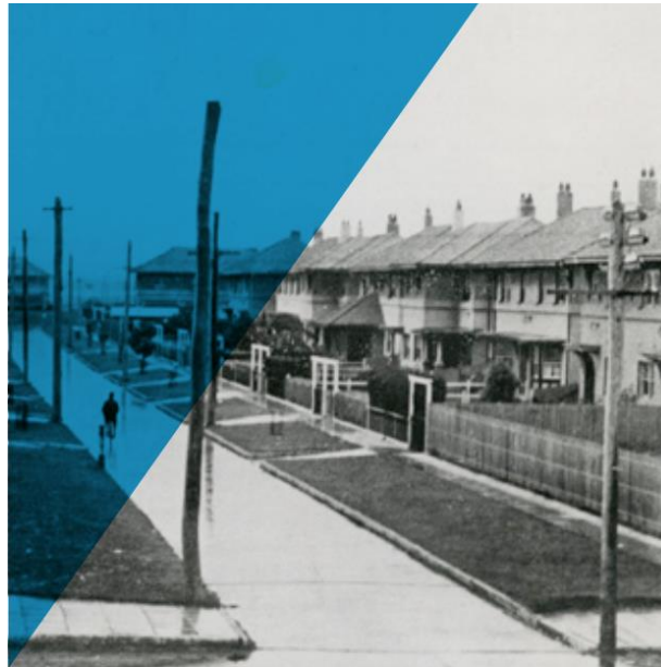
First houses built at Fishermans Bend sponsored by State Savings Bank of Victoria, 1930-1939. Port Phillip City Collection
