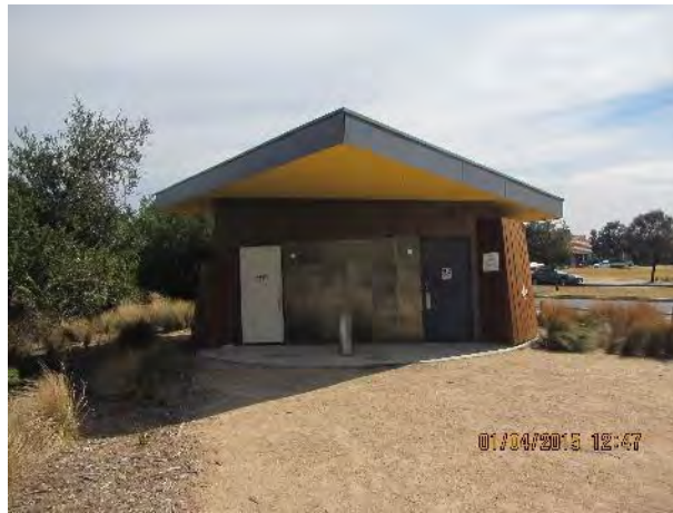
Figure 10. Sandridge Foreshore amenities block
