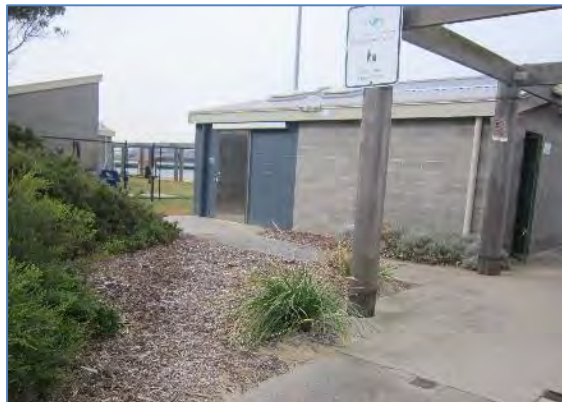
Figure 9. Womens amenities block at Sandridge Foreshore
