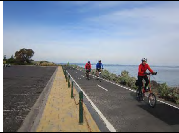
MO1 looking south
