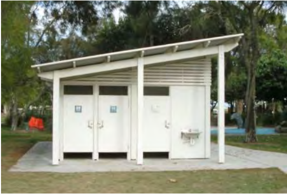
Figure 13. An example of an amenities block with good design features to promote safety (Brisbane City Council 2013).
