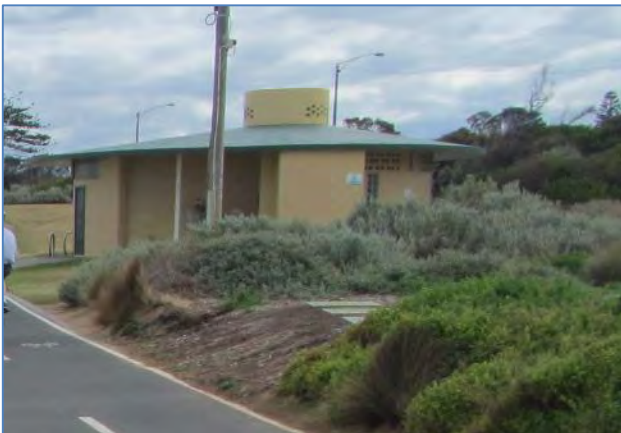
Figure 11. Point Ormond amenities block looking from the east
