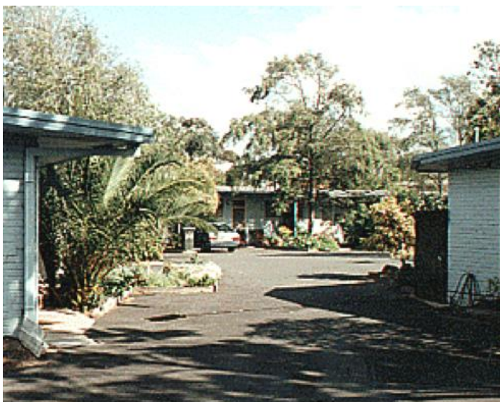
Figure 3 - The flats c.1990s prior to the alterations carried out in 2000 (Source: City of Port Phillip)
