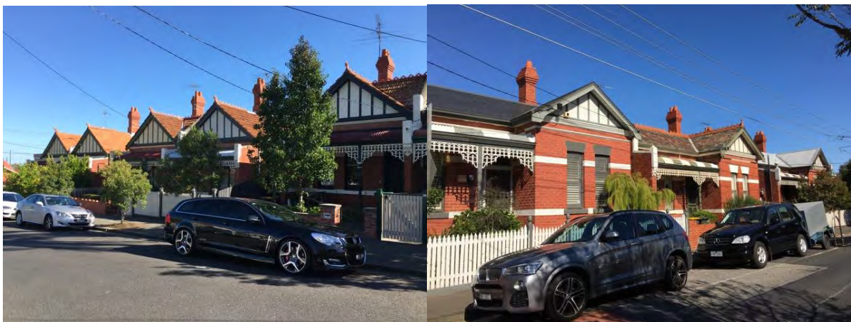
Figure 6.10–14 – Edwardian houses in Lambeth Place (left) and Octavia Street (right)
