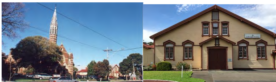
Figure 6.10–8 – St. George's Uniting (former Presbyterian) church of 1877-80 and the former St. Kilda Orderly Room dominate the Chapel Street hill
