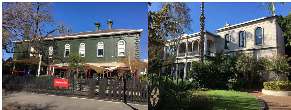
Figure 6.10–10 – The former 'Marlton' (left) and 'Rondebosch' (right), both now part of St Michael's Grammar School.
