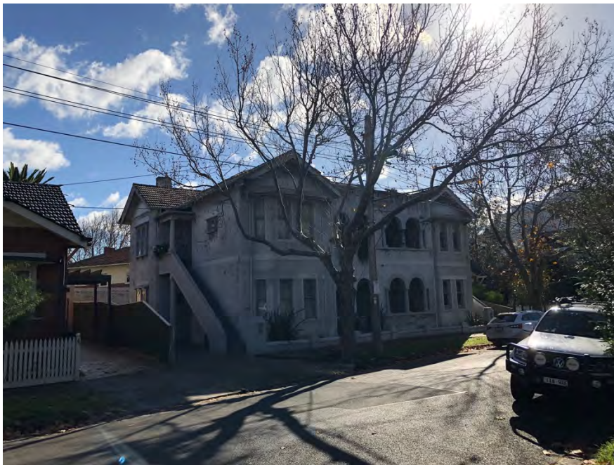
Figure 2: Early twentieth century flats on the northwest side of Tiuna Grove currently within the HO8 Elwood: Glenhuntly and Ormond Roads heritage overlay.
