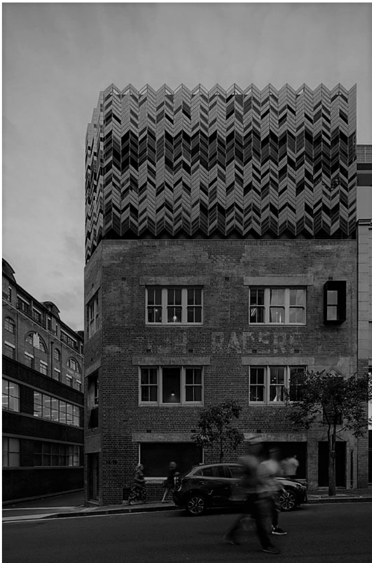
Photo 12. Designed by Breathe Architecture, the Paramount Hotel in Surry Hills, New South Wales is a good example of using lightweight materials to provide a contrast with the solidity of the original masonry building. The colour and chevron patterning of the copper screen provide a contemporary reference to the original brickwork and also provide shade and natural ventilation (image: Sharyn Cairns)
