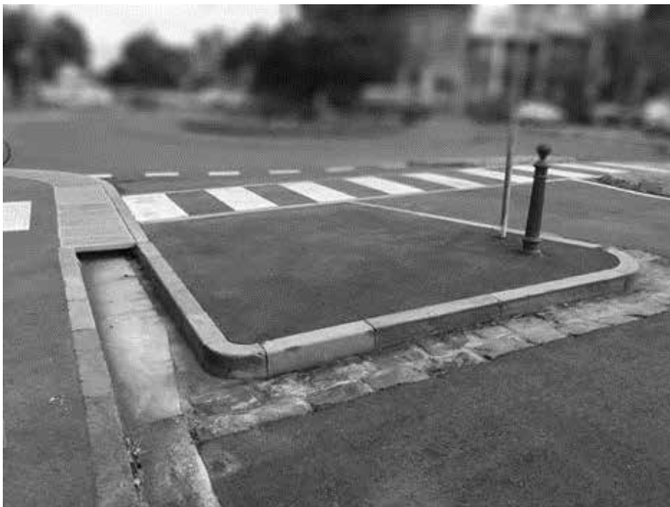
Photo 23. The installation of this new kerb outstand and associated pedestrian crossing in Bank Street, South Melbourne uses sympathetic materials and also ensures that the historic alignment and layout of the original kerb and channel remains evident.
