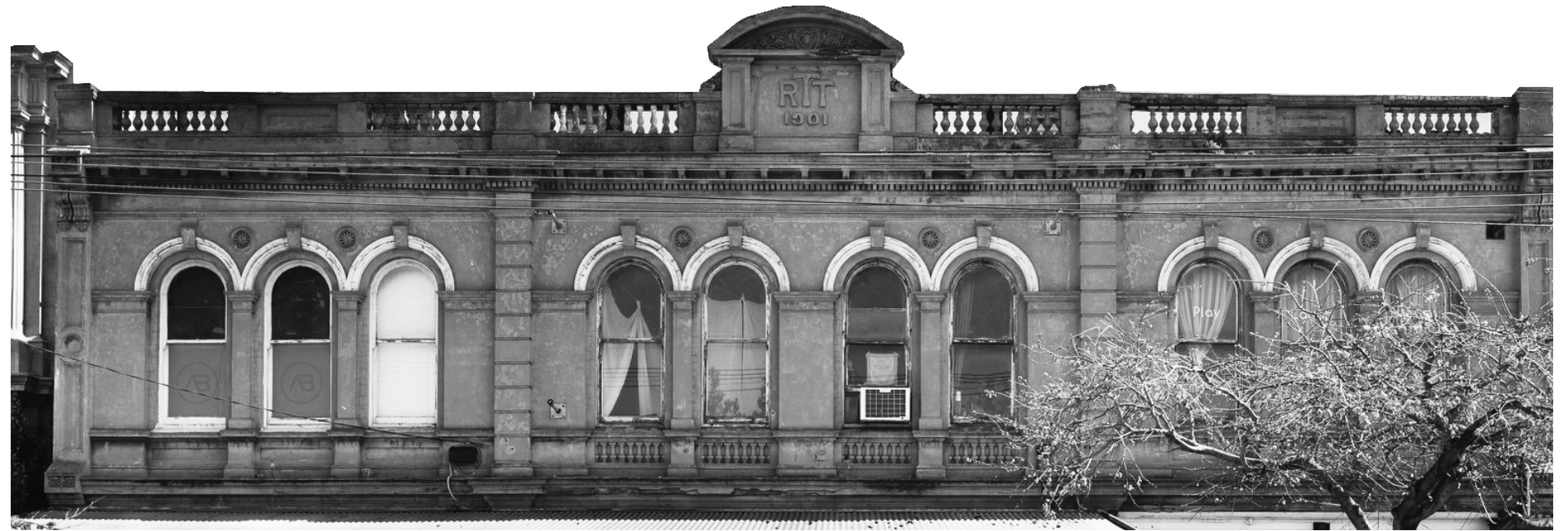
Existing Heritage Facade at 146-150 Bridport Street
