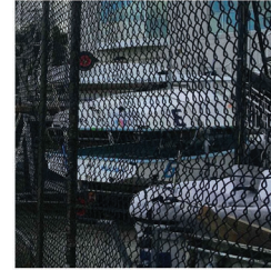
F06 BLACK CYCLONE MESH Existing cyclone mesh defining the perimeter of the yard in west, north and south elevations
