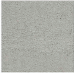
F02 GRAY RENDERED WALLS External brick walls on east elevation covered with gray render (darker shade than F01)
