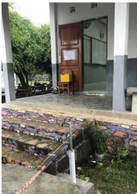
Taps have been installed in the front of all school buildings.
